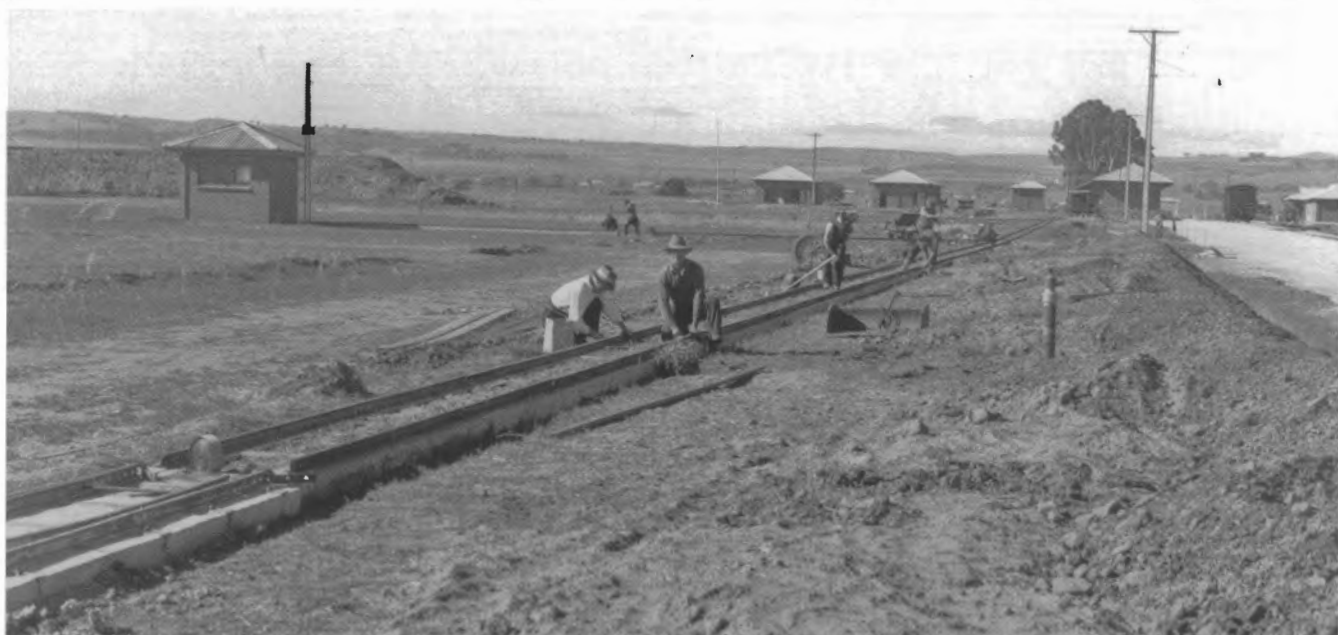
Construction activities on the northern 'main line', May 1941, with an Engineering and Water Supply Department 'Dobbin' side-tipping truck visible behind the workers. Photo: SA Water
