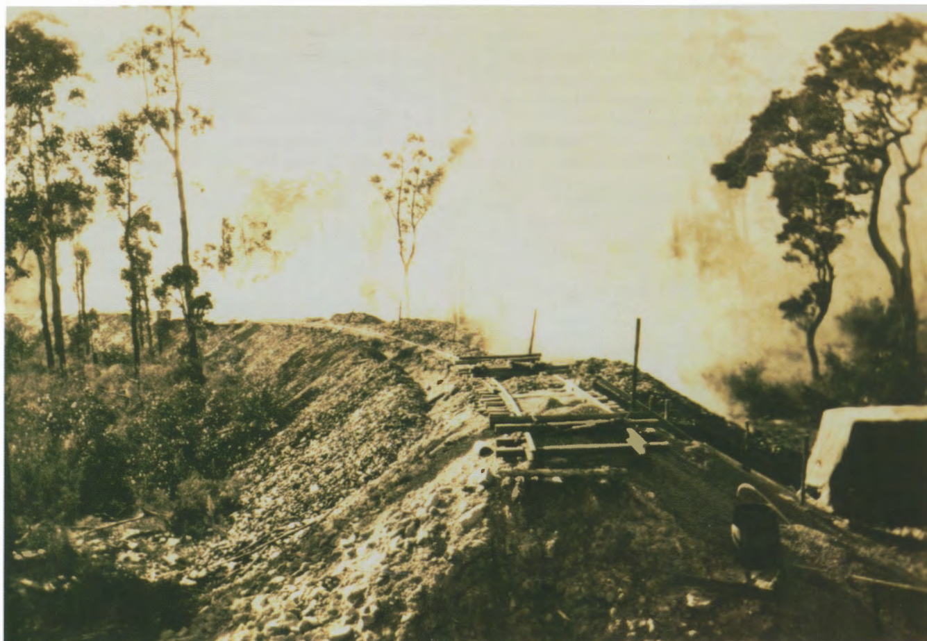
In May 1927, chitter (coal waste) is being burnt on-site to form a consolidated clinker, which will then be used to augment the earth filling of the embankment.
