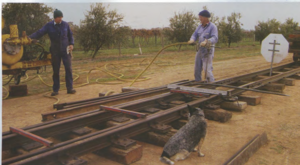
The Cobdogla Steam Friends track crew installing a passing loop near the half way mark on the track extension to Loveday using turnouts obtained from the Loxton Station yard. Robbie Osborne is turning on the air at the compressor and Gary Wright is about to drill some holes, while 'Cody', the works supervisor, looks on in the foreground. Photo: Denis Wasley
