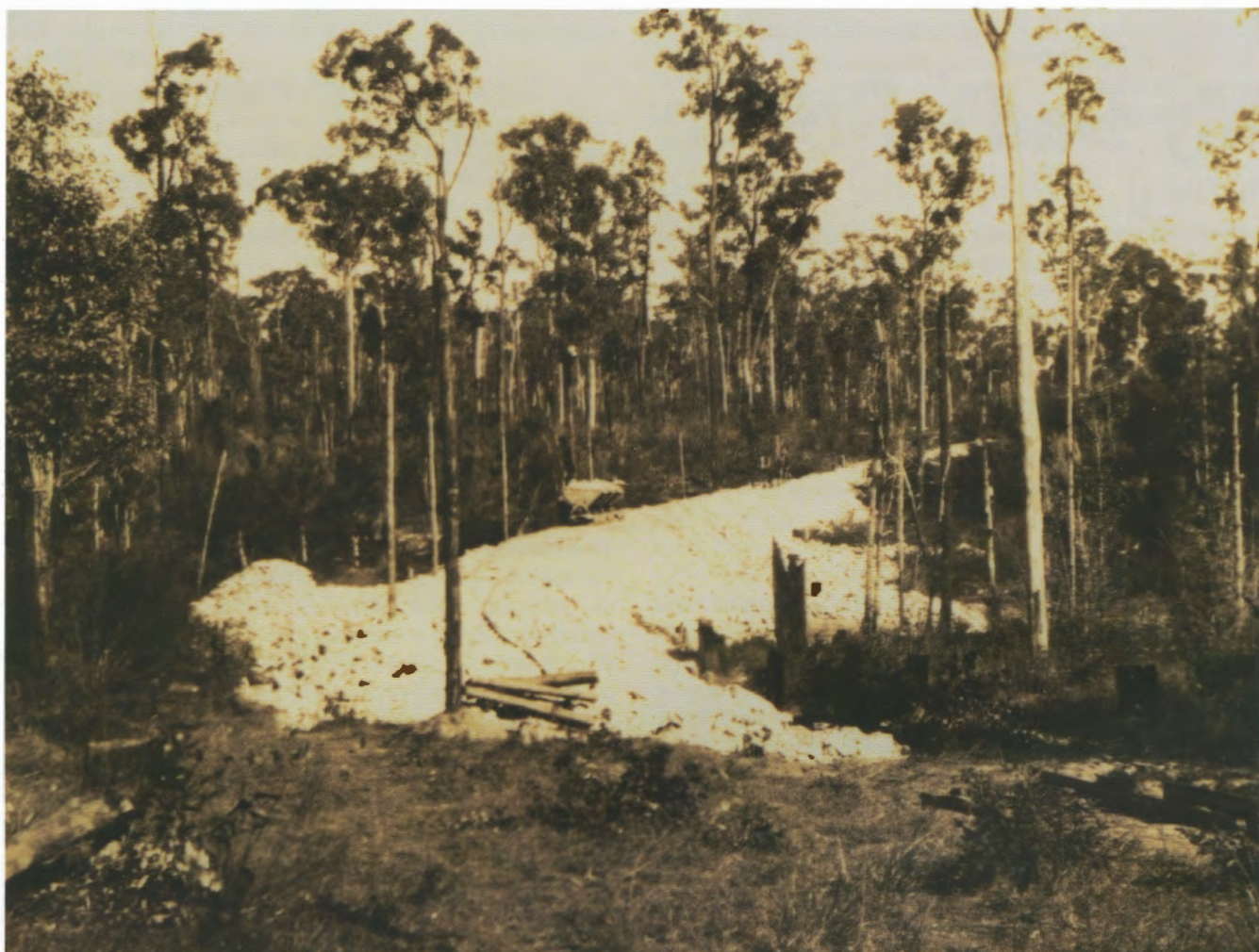
Building the second railway bank using side-tipping skips, May 1927.
