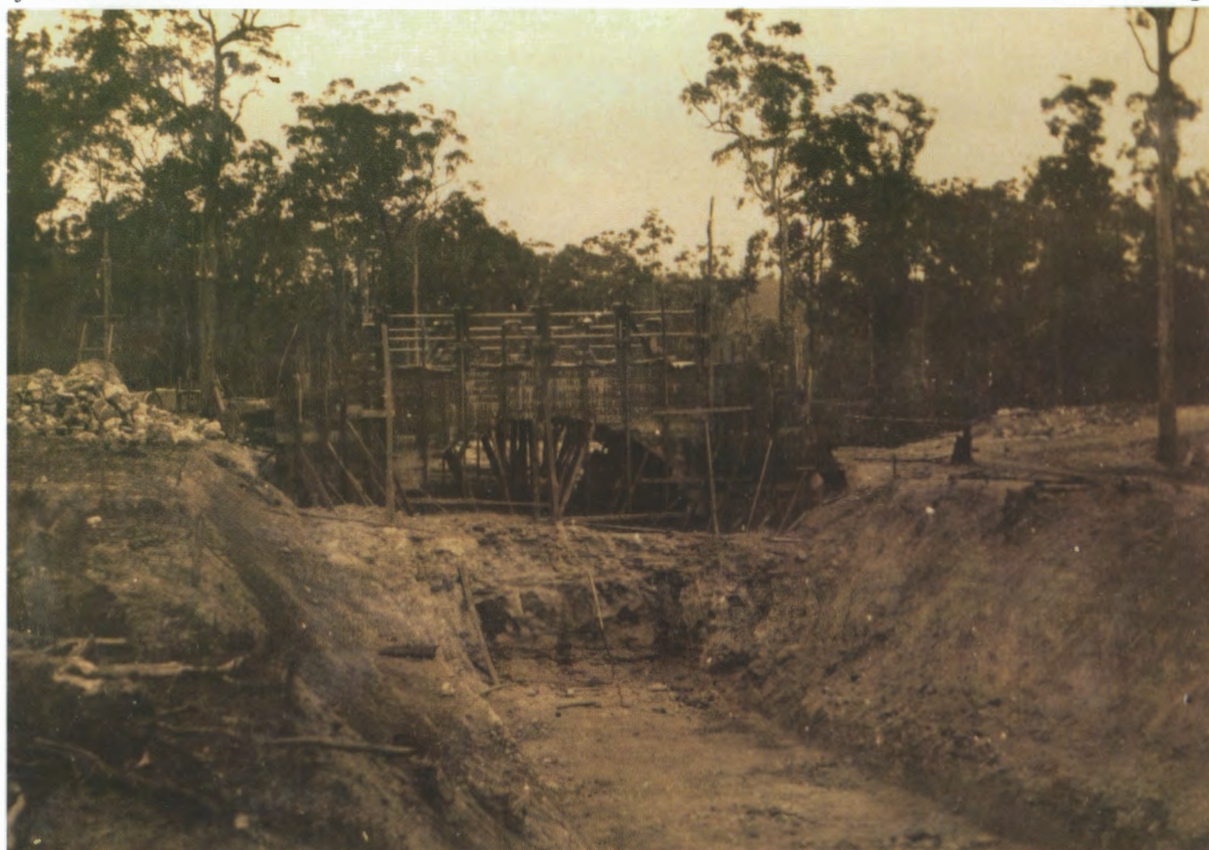
On 8 December 1927, the forming of the Lake Road Bridge is seen in position.
