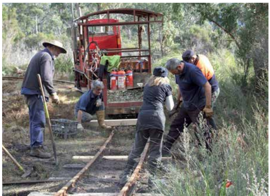
Left: Extensive track upgrade work is currently being undertaken on the Ida Bay Railway with the aid of machinery.. Right: Spot sleeper replacement on the railway is another matter – all hands on work.
