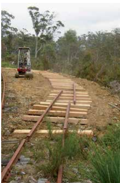
Left: Extensive track upgrade work is currently being undertaken on the Ida Bay Railway with the aid of machinery.. Right: Spot sleeper replacement on the railway is another matter – all hands on work.
