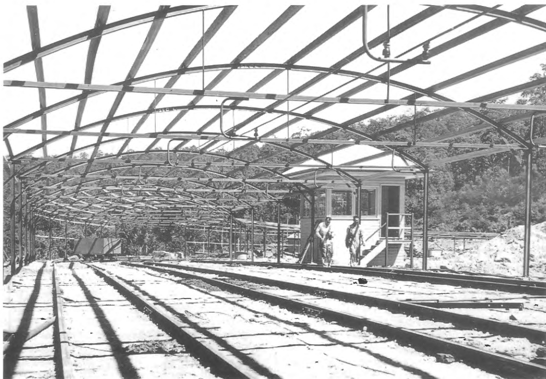
Construction of the trolleywire system around 1954. This scene shows the area leading up to the dump hopper before being roofed over, with only the centre track electrified. The traffic officer cabin is on the right.
