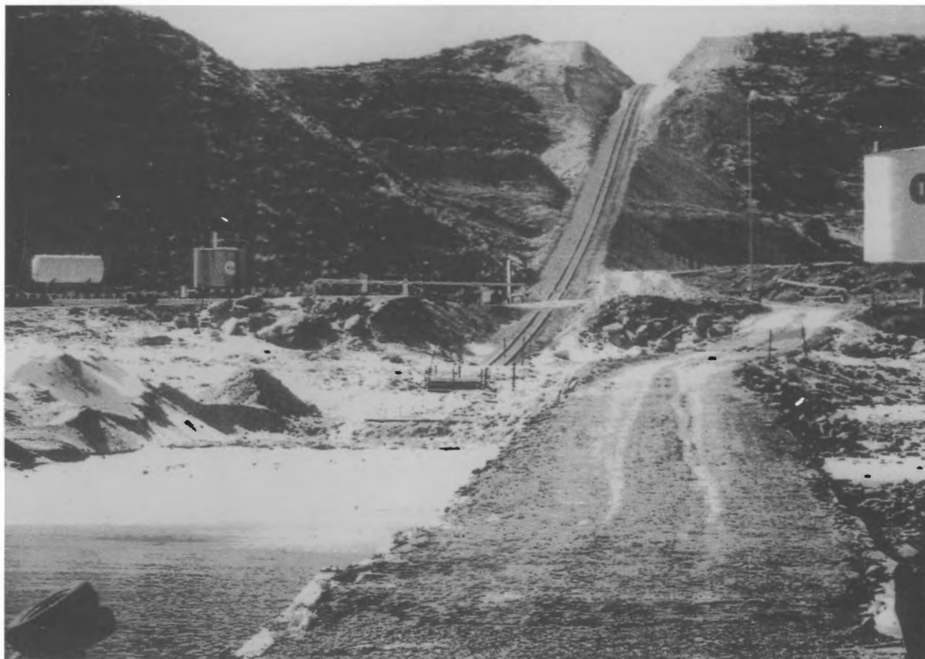
The second light railway, built to deliver a 2050 metre long extension to the existing undersea pipeline, is seen under construction in early 1992.
