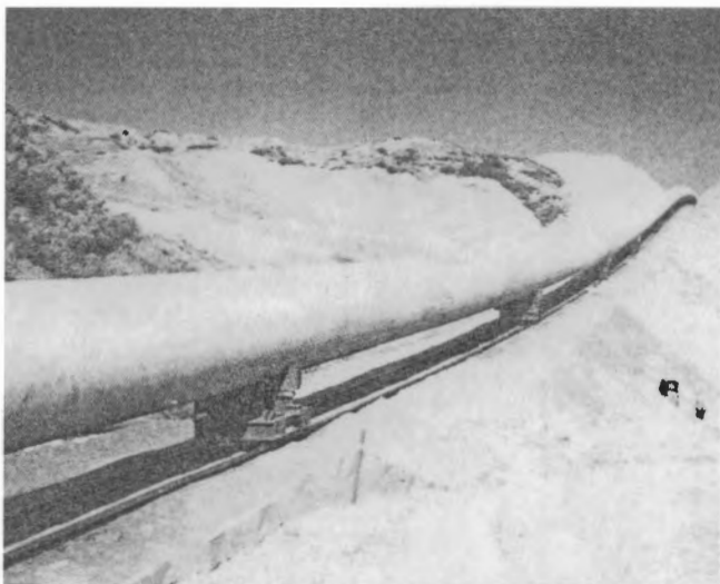
At the cliff-top end of the railway, a section of pipeline sits on its 4-wheeled trucks, waiting to be lowered down the escarpment. Photo: P Dwyer
