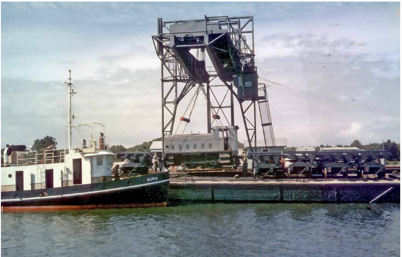
Above: One of the two 28-ton Ruston & Hornsby DM 0-4-0 diesel locomotives at the head of a rake of loaded stone trucks at Iluka. The 10-ton steam crane's anchor beam crosses the railway behind the trucks and beyond that is the superstructure of the 40-ton electric derrick crane. The rails ahead of the locomotive continue onto the northern breakwater where the load will be deposited. Photo: Maclean District Historical Society Below: Transferring the Ruston & Hornsby diesel locomotive and the stone truck fleet between Yamba and Iluka was done on at least four occasions as construction activity switched between the north and south breakwaters. Here the 40-ton Yamba gantry crane is lifting the locomotive off the stone punt which brought it across from Iluka. A row of chained-down stone trucks await their turn. Photo: Norman Brown collection
