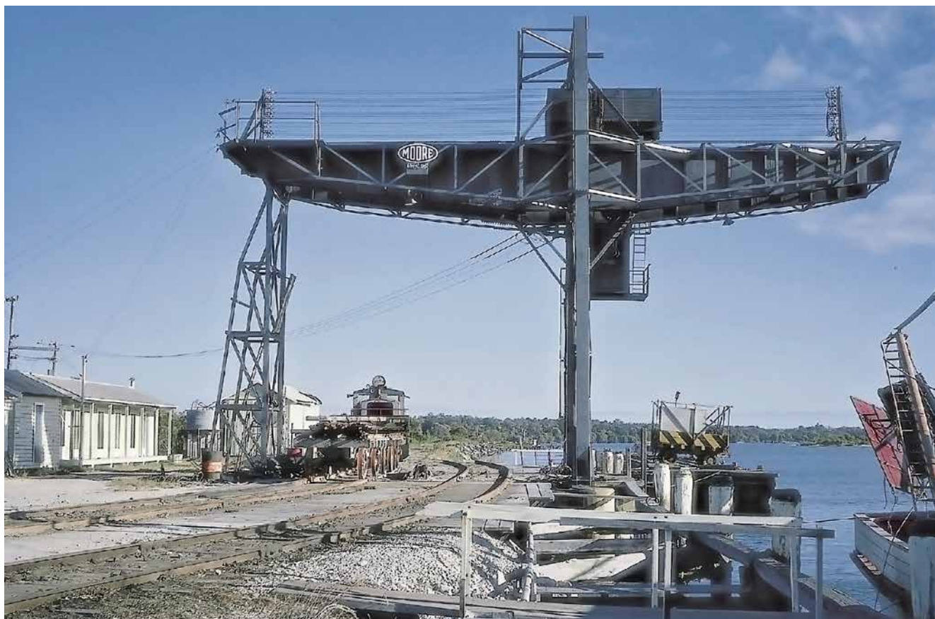
A 40-ton electric portal crane was erected on the Yamba Crane Wharf in 1956 to handle concrete blocks produced at Ilarwill Quarry. There was no stock-piling facility, and blocks lifted off punts were placed onto waiting stone trucks to be taken directly to the southern breakwater tip site two miles down-river.
