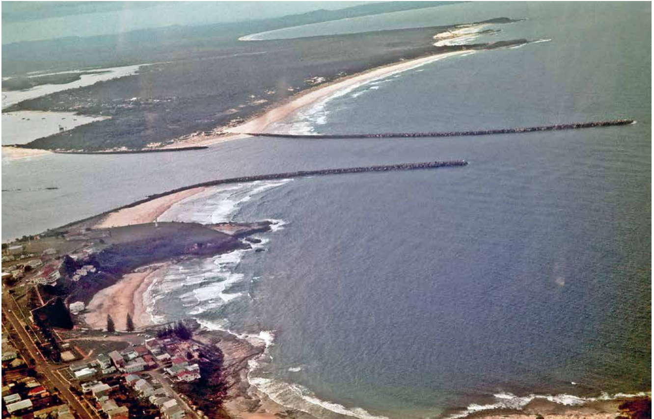
An aerial view of the Clarence River entrance taken after both breakwaters had been completed to their authorised limits in July 1968. The unequal lengths diffused the tidal flows, which were then insufficiently focused to maintain the desired 20ft channel depth across the off-shore bar. This was remedied by extending the South Breakwater to same length as the North, which required another three years' work. Photo: Norman Brown collection
