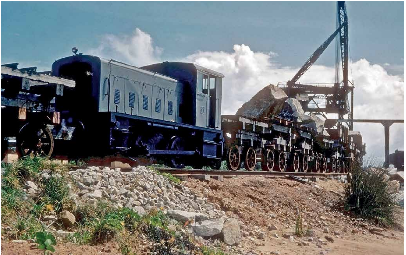
Above: One of the two 28-ton Ruston & Hornsby DM 0-4-0 diesel locomotives at the head of a rake of loaded stone trucks at Iluka. The 10-ton steam crane's anchor beam crosses the railway behind the trucks and beyond that is the superstructure of the 40-ton electric derrick crane. The rails ahead of the locomotive continue onto the northern breakwater where the load will be deposited. Photo: Maclean District Historical Society Below: Transferring the Ruston & Hornsby diesel locomotive and the stone truck fleet between Yamba and Iluka was done on at least four occasions as construction activity switched between the north and south breakwaters. Here the 40-ton Yamba gantry crane is lifting the locomotive off the stone punt which brought it across from Iluka. A row of chained-down stone trucks await their turn. Photo: Norman Brown collection
