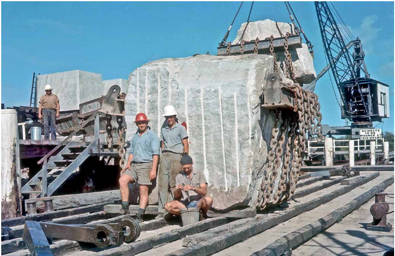
The lifting gear used on large stone blocks weighed two tons which limited the maximum block weight to 38 tons to enable them to be handled by the 40-ton cranes at Ilarwill, Iluka and Yamba. This block on the deck of a punt at Iluka shows the pattern of holes bored one foot apart with a jackhammer and loaded with cordex to shape it into the required 8ft by 7ft size. Photo: Norman Brown collection
