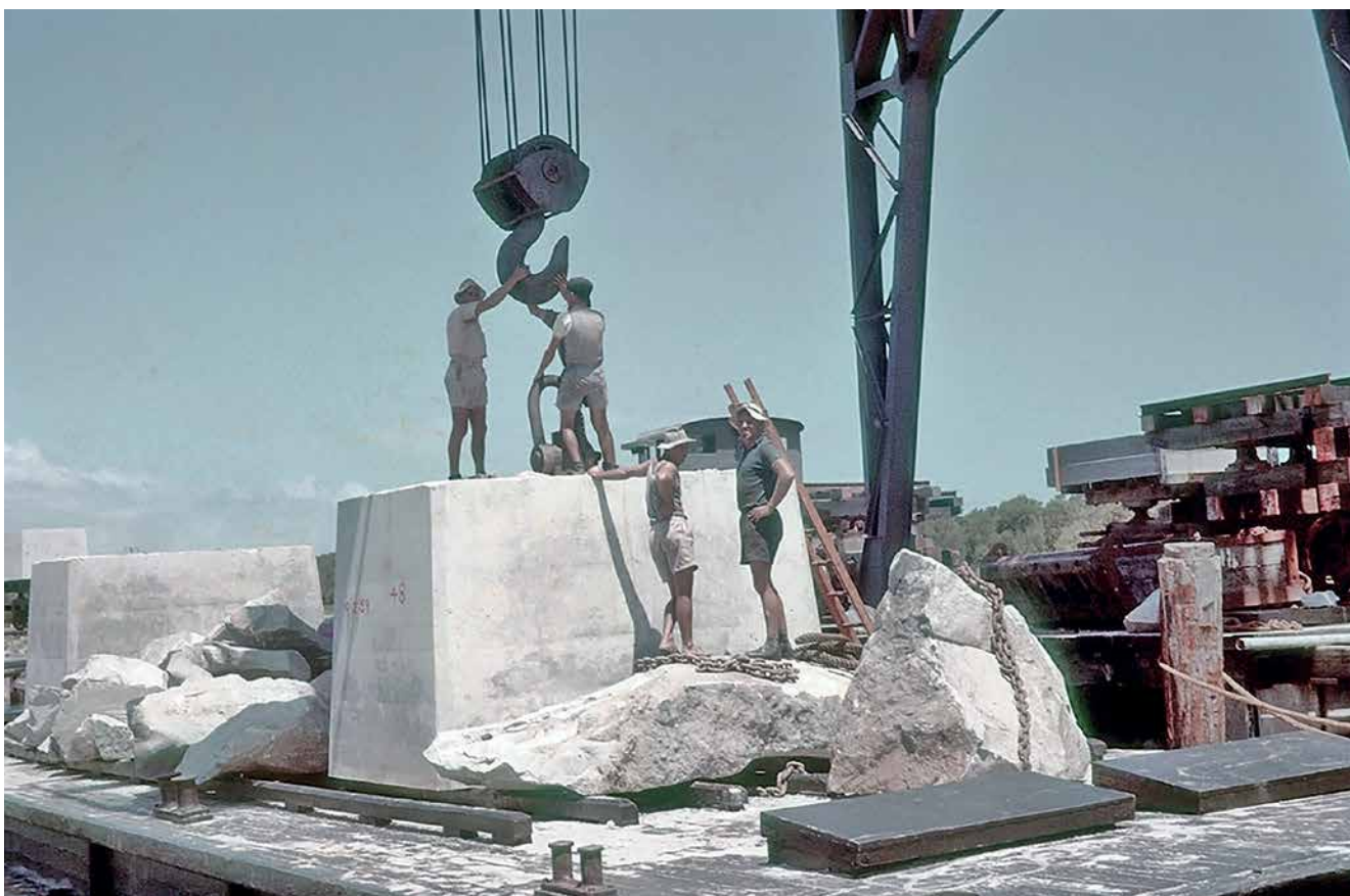
Below: The 40-ton electric crane at Iluka Crane Wharf prepares to lift a concrete block from the deck of a punt to a waiting rail truck on the wharf, with the cab of the diesel locomotive visible behind. A shackle was screwed into the top of each block prior to lifting. A more relaxed attitude to OH&S prevailed at that time. Photo: Norman Brown collection
