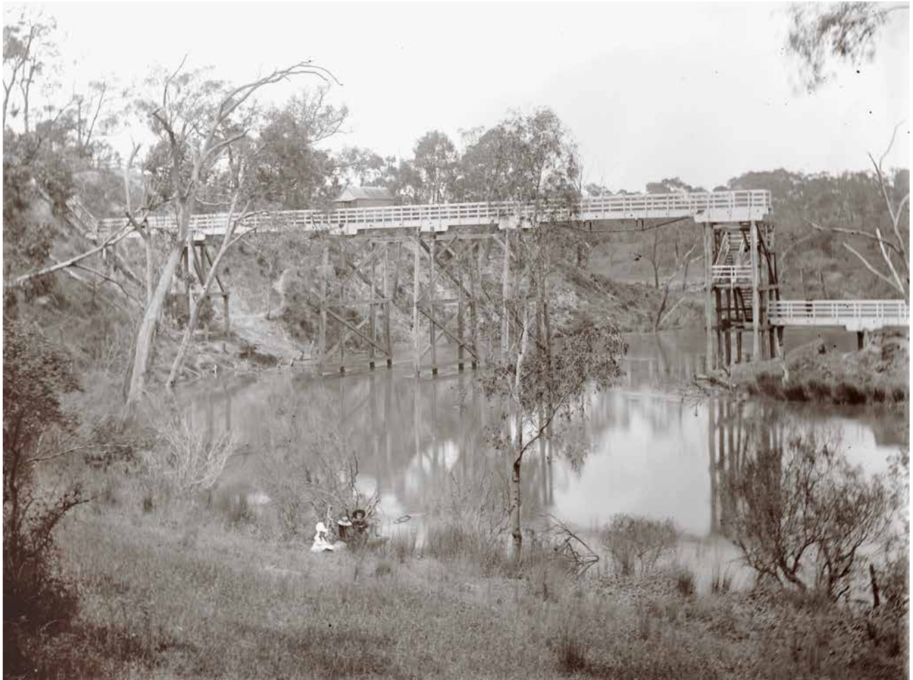
Zig Zag Bridge viewed from upstream. The central pier and substructure was removed in 1910 and replaced with a single span similar to those near the banks. State Library Victoria image H83.94/416
