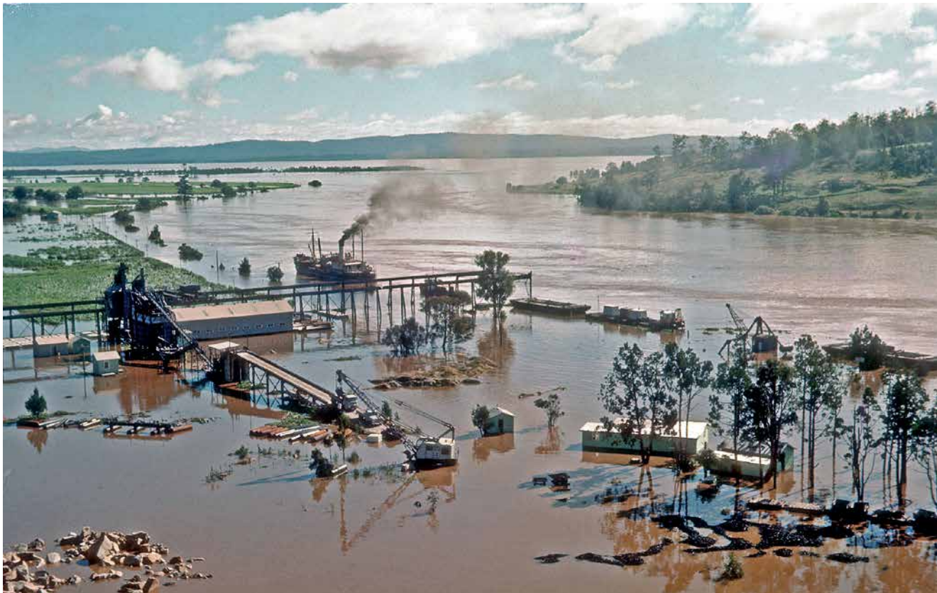
The May 1963 Clarence River floods inundated Ilarwill Quarry and its concrete block plant, halting production for several weeks. The pre-flood line of the river bank is marked by the dredge H.E. Street, the tugboat Iluka, the row of stone punts and the 10-ton steam crane. The extent of the elevated 40-ton crane gantry can be appreciated in this photograph.
