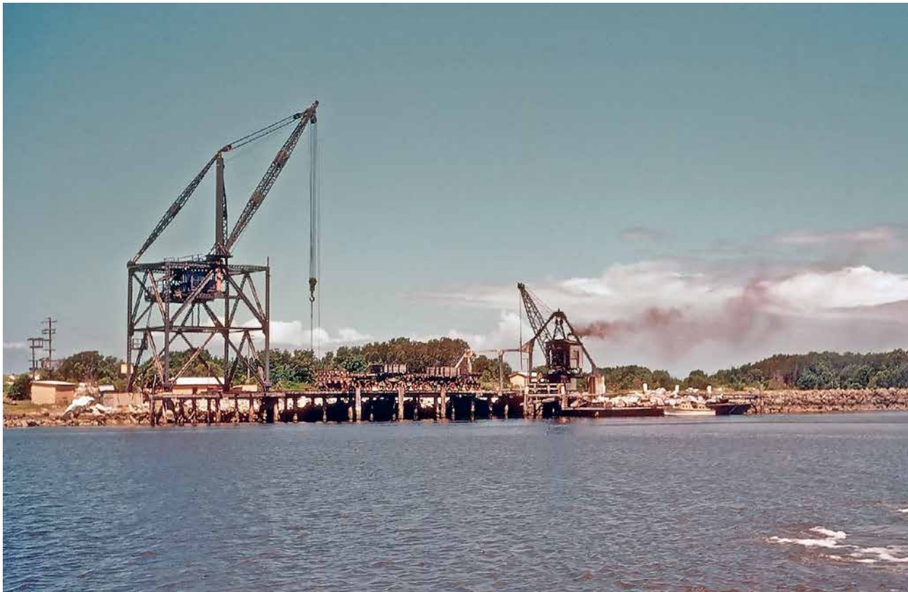
Above: Two cranes operated on the Iluka Crane Wharf; a 10-ton steam crane installed in 1951 and a 40-ton electric derrick crane commissioned in 1959. Stone embankments and wooden wharves supported the river front railway siding where the cranes loaded stone boulders and concrete blocks onto rail trucks for the short trip to the north breakwater construction site. Photo: Norman Brown collection
