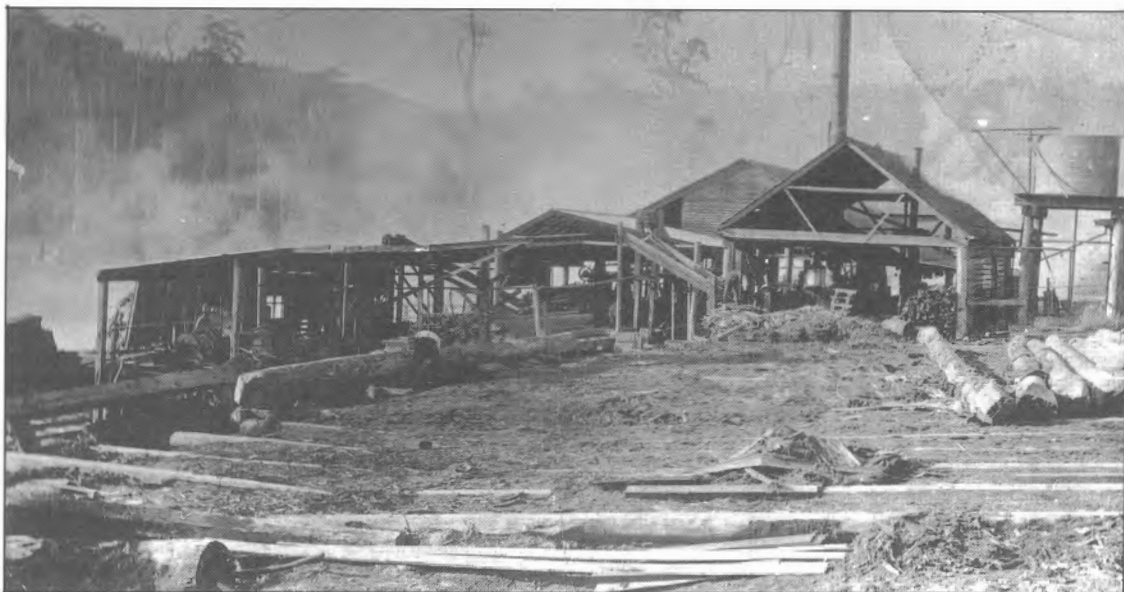
View of the south-west end of the Pines & Hardwoods sawmill at Simsville, c.1924
