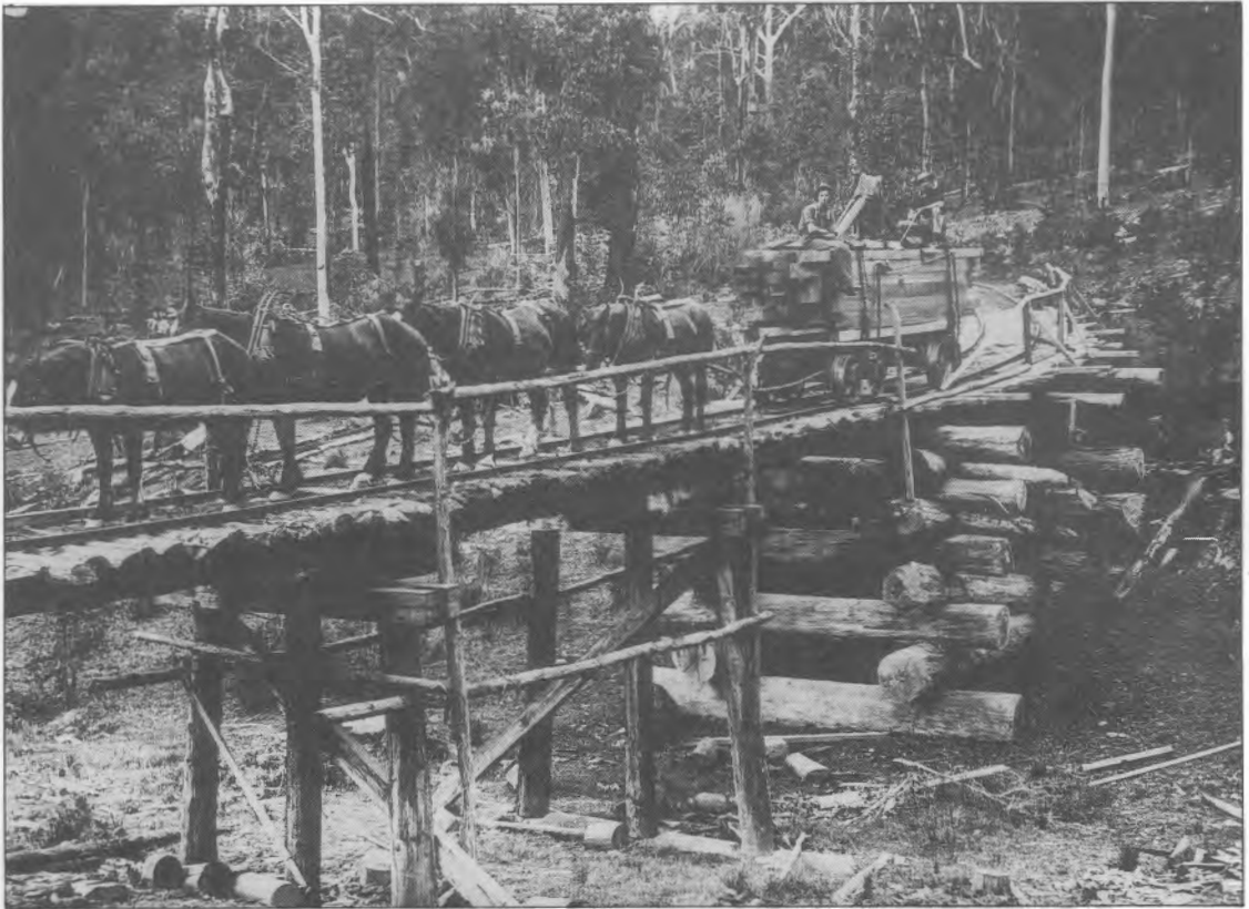
A small trestle bridge near the Jarrah Mill on Millars' horse tramway, c.1913
