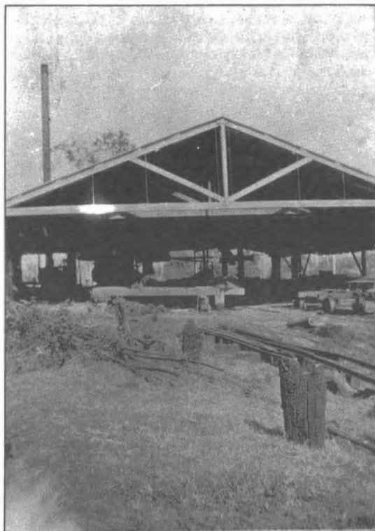
The new Smith & Ellis Jarrah mill at Simsville in 1936. Charred posts in the foreground may be part of the fire-destroyed Pines & Hardwoods mill.
