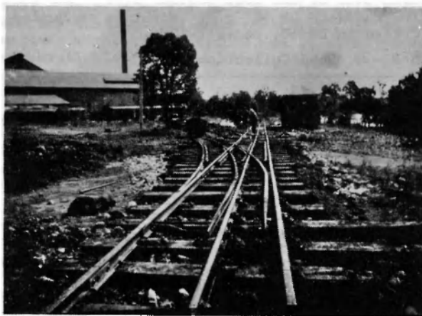
Top - Dual gauge (2-ft. and 3-ft.6-in.) points at Isis Central Mill. Photo - G. Bond coll'n.
