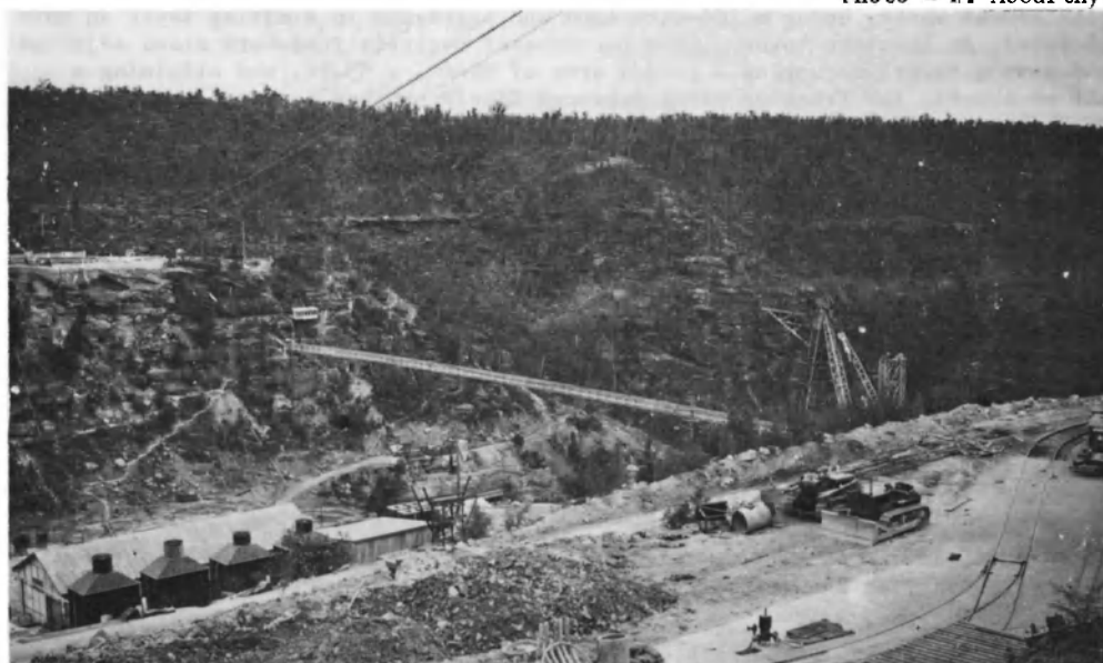
Below - Warragamba dam site showing the suspension foot bridge, and standard and 2-ft. gauge track on the lower right. 23rd. October 1954.
