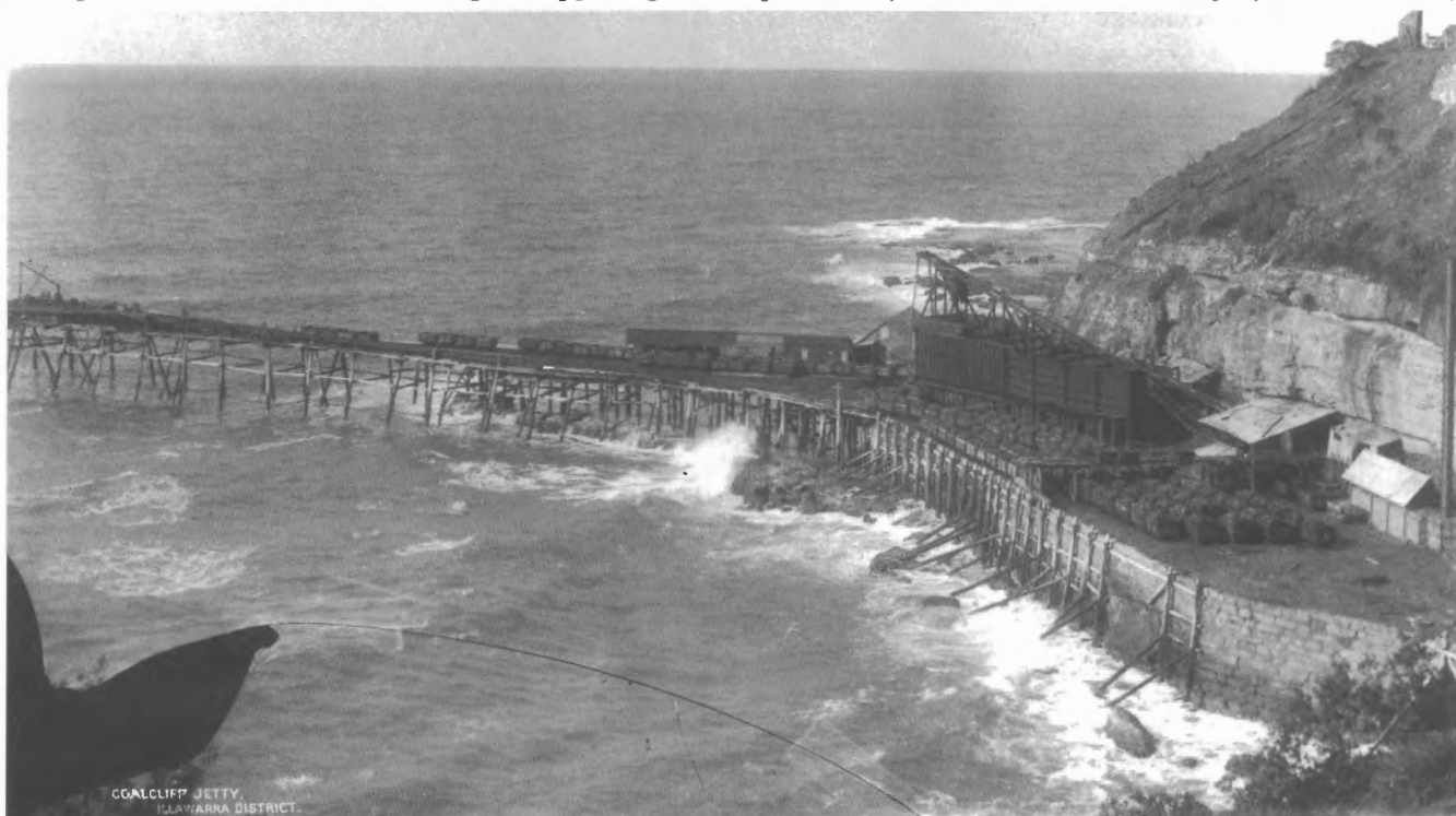
The third Coal Cliff jetty, seen in 1898. A large rock-faced working platform has replaced the original timber trestle arrangement.
