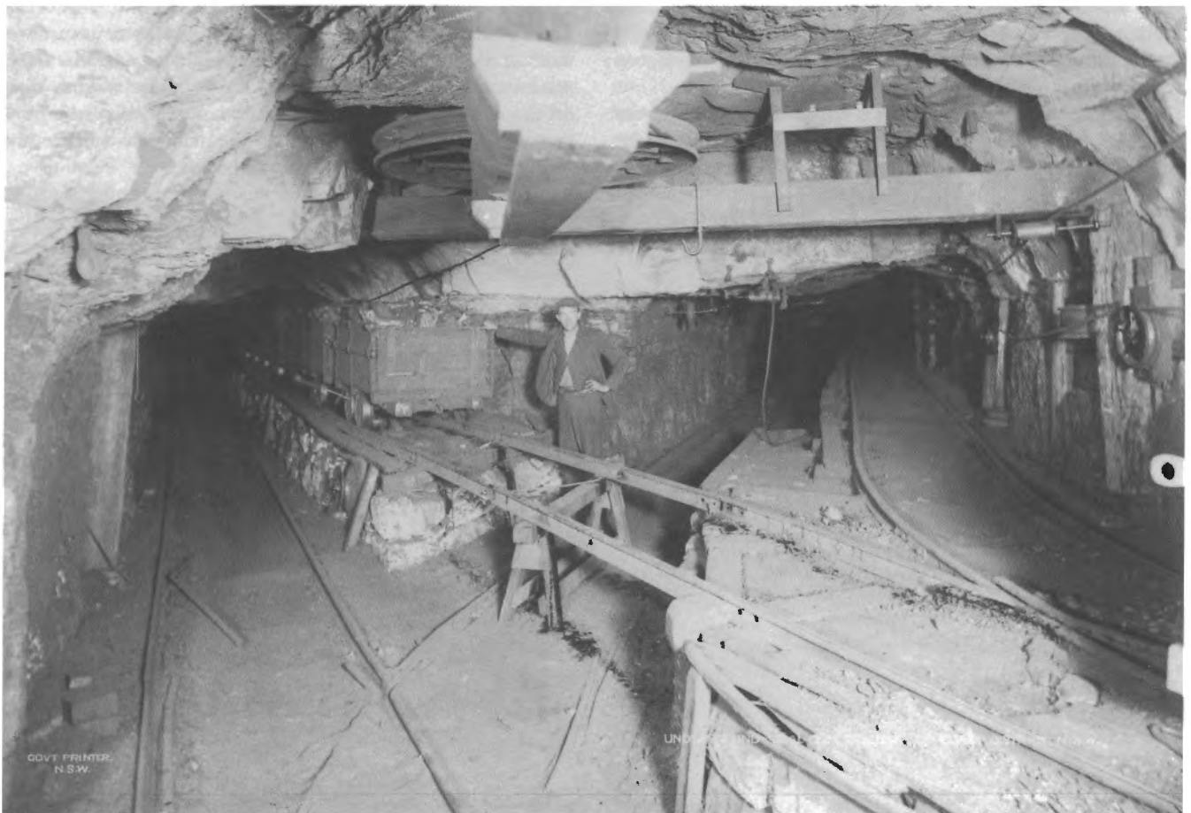
Looking into the mine. The tunnel straight ahead led to the western district and that on the right to the northern district. The return line to the north is shown cutting through the line bringing coal from the west.
