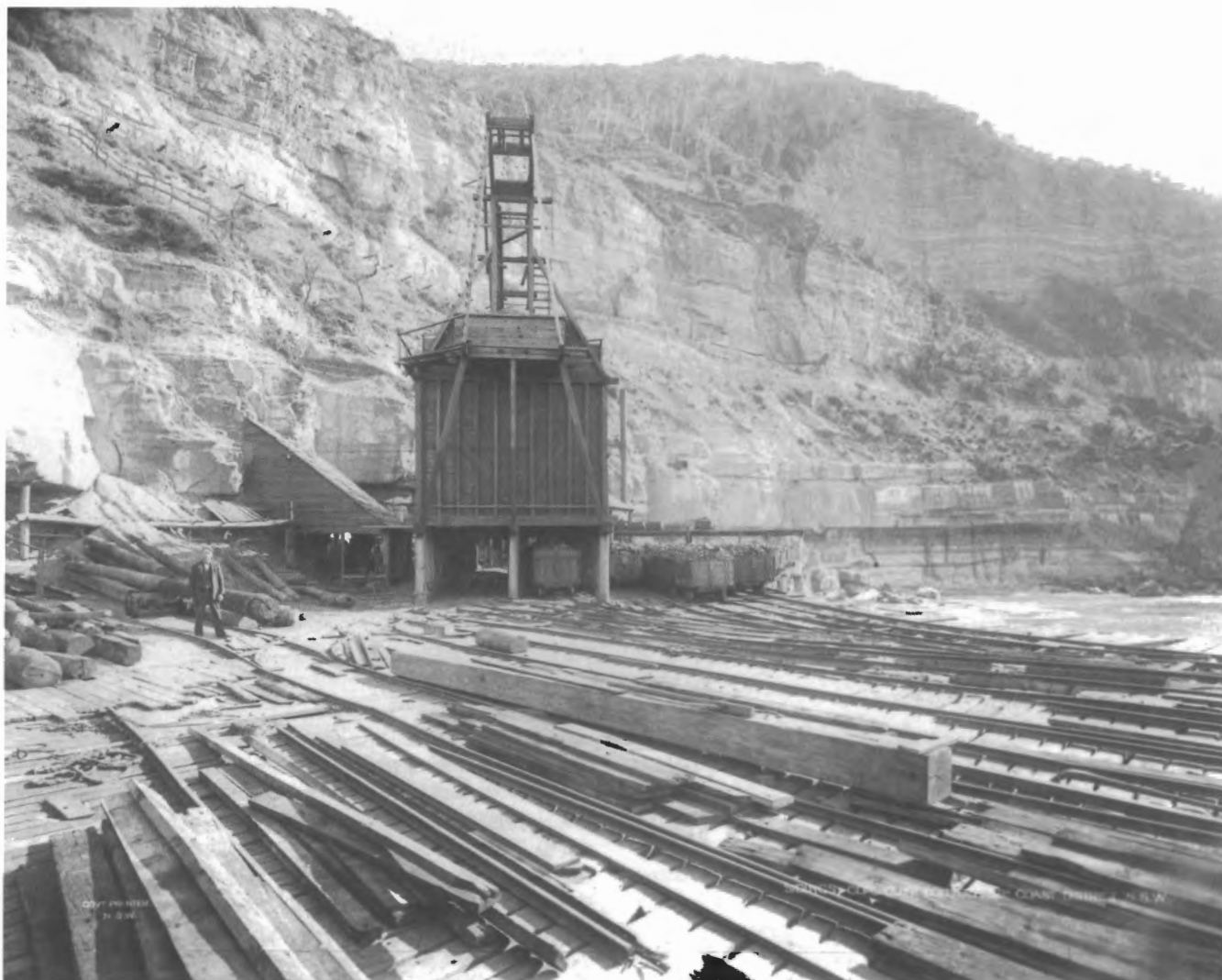
Round poles, hewn baulks of structural hardwood and spare rail littered the cramped deck of the jetty. The storage hopper for slack coal is in the background.
