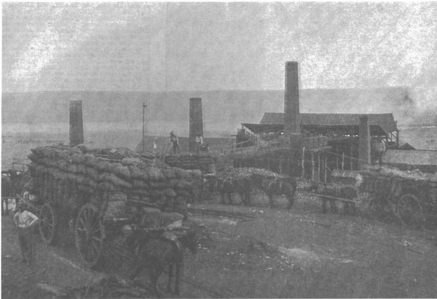
Teamsters deliver bagged coke to the water jacket furnaces at Nymagee in 1902. The old reverberatory furnaces are on the right. The Sydney Mail, 2 Nov 1902
