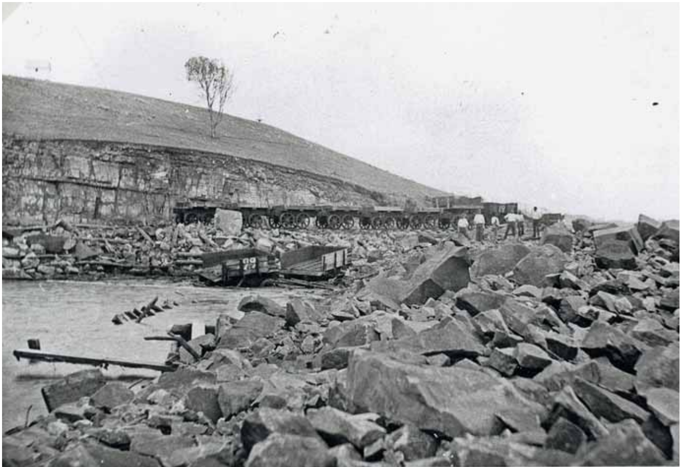
Stone trucks stand on the breakwater railway line at the foot of Flagstaff Hill, Harrington as labourers work to retrieve trucks swept off the training wall during the May 1898 Maitland Gale. The side of the hill was cut back to make room for the railway.
