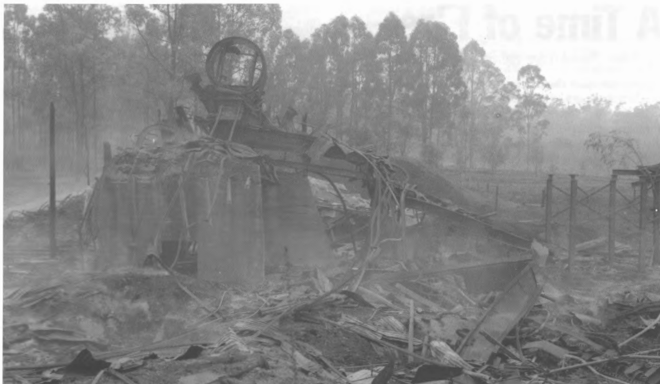
Above: The remains of Millfield Colliery screens after the November 1968 fire. The circular object atop the concrete foundation is the skip tumbler. Left: Some we saved! Coal wagons smoulder on Maitland Main sidings after the fire. Below: And some were Lost! Burnt-out wagons on Millfield Colliery sidings, November 1968.
