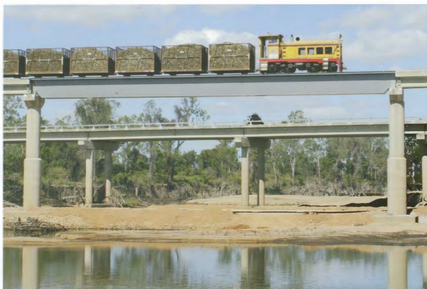
On 5 July, Inkerman Mill's EM Baldwin B-B DH IYAH (6558.1 6.76 of 1976) eases its train across the temporary span of Invicta Mill's Landers Creek bridge in remote control mode pending approval for manned crossings to be made. Photo: Scott Jesser
