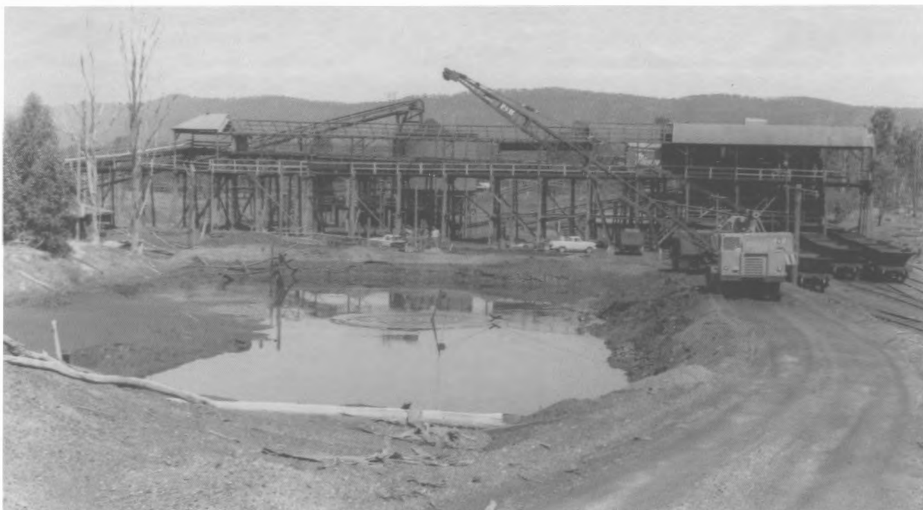
Maitland Main Colliery Pit Top. The dragline is cleaning out the washery sludge pond. To the right, empty wagons wait to be gravitated under the screens for filling. December 1967
