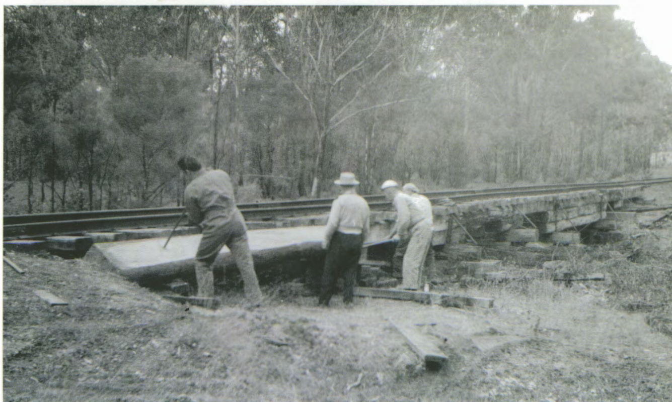
Maintenance work on No.1 Bridge Maitland Main Colliery branch. The wagon repairers, carpenter and fitter bar a new longitudinal bearer in place in October 1969
