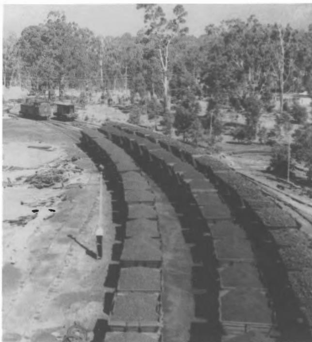
Full Coal Standage Maitland Main Colliery. The locomotive has set off the van and is about to back onto a loaded train. Note the two roads of small coal.
