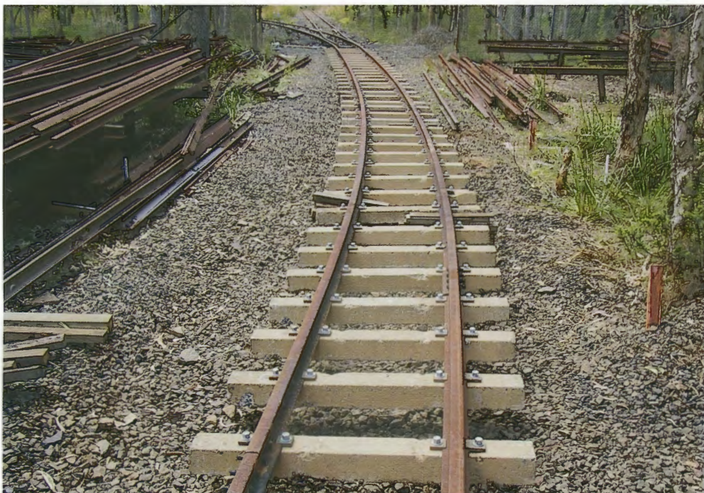
A section of recently laid track at the Illawarra Train Park in August 2008 which utilises concrete sleepers from Queensland sugar mills.
