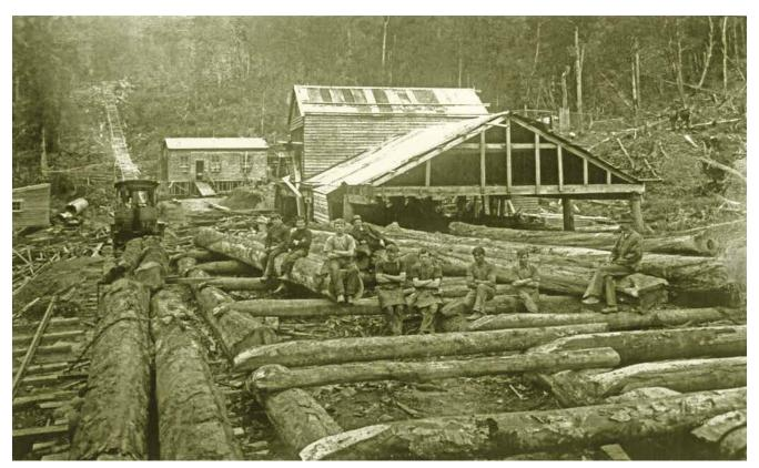
Watson's Charming Creek Mill circa 1917. A steam locomotive has recently arrived with a rake of logs for the mill. Beyond the locomotive is the abandoned incline from the original outlet tramway, while the new line down the Ngakawau gorge curves off to the left. The mill crew is posed for the photograph, with Bob Watson reclining on the logs behind them. The solitary figure seated on the log on the far right is Murdoch McDonald. DoC interpretive material, Charming Creek Walkway.
