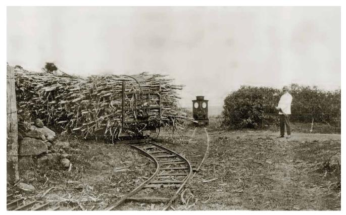
Krauss locomotive in the cane fields at Cudgen. Note the 'jump points' in the foreground in front of the cane wagon.
