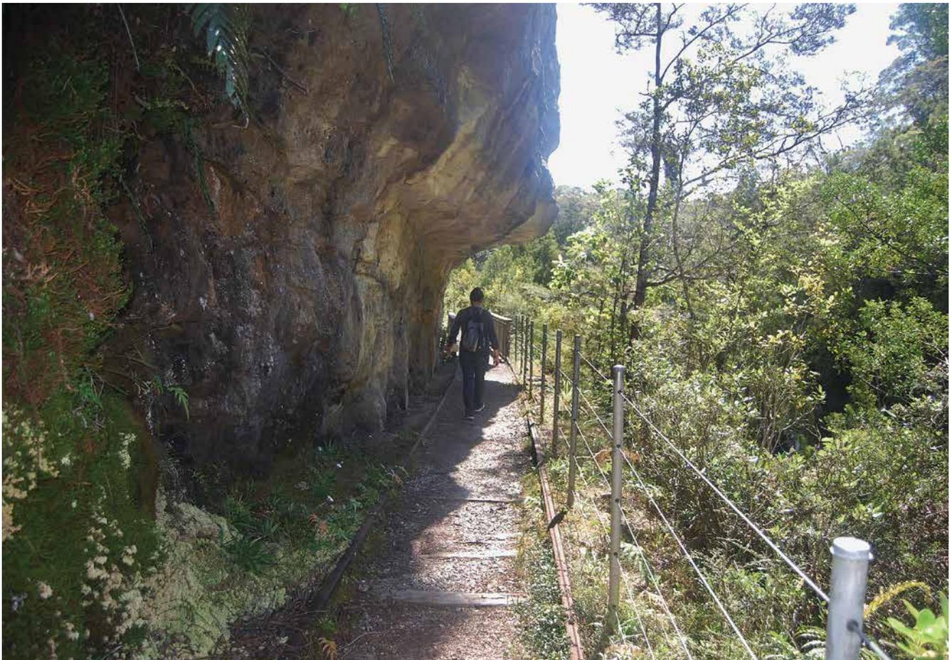
*'The Verandah', a section of tram close to the Charming Creek mill which had to be blasted out of the cliff face. Just outside the modern DoC fence, the cliff face drops sheer to Charming Creek.*
