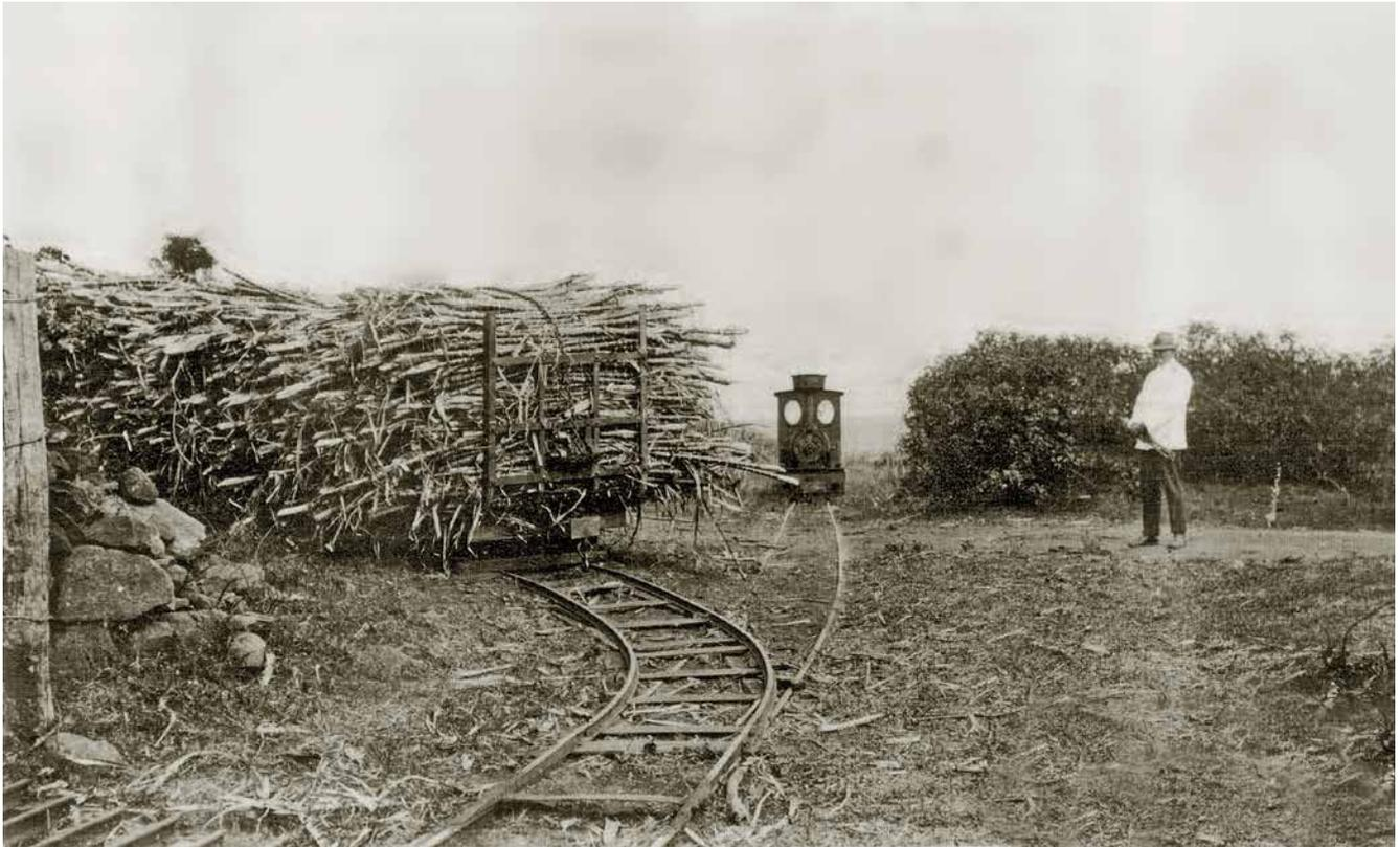
Krauss locomotive in the cane fields at Cudgen. Note the 'jump points' in the foreground in front of the cane wagon.
