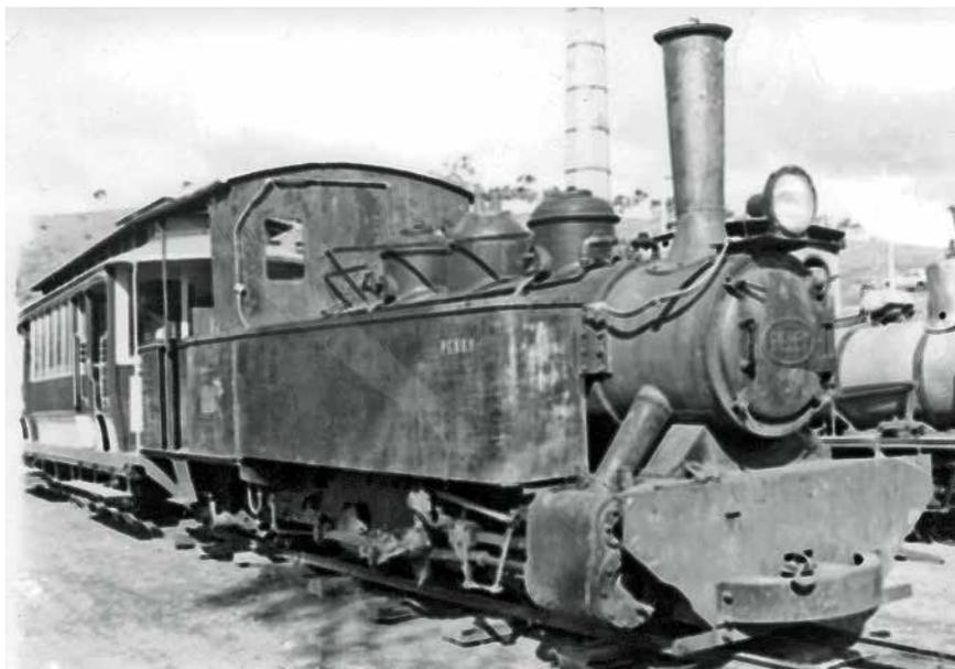
Ex Bingera Perry at Goulburn in late 1976 with the ex Sydney tramways 'D' Class four wheel car which Bruce Macdonald rebuilt on a pair of ex North East Dundas Railway bogies. It has now been restored to its authentic form at the Sydney Tramway Museum. Photographer Unknown
