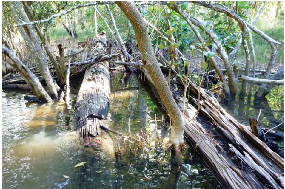
Bridge stringers in Poundyard Creek. Photo: Ian Barnes
