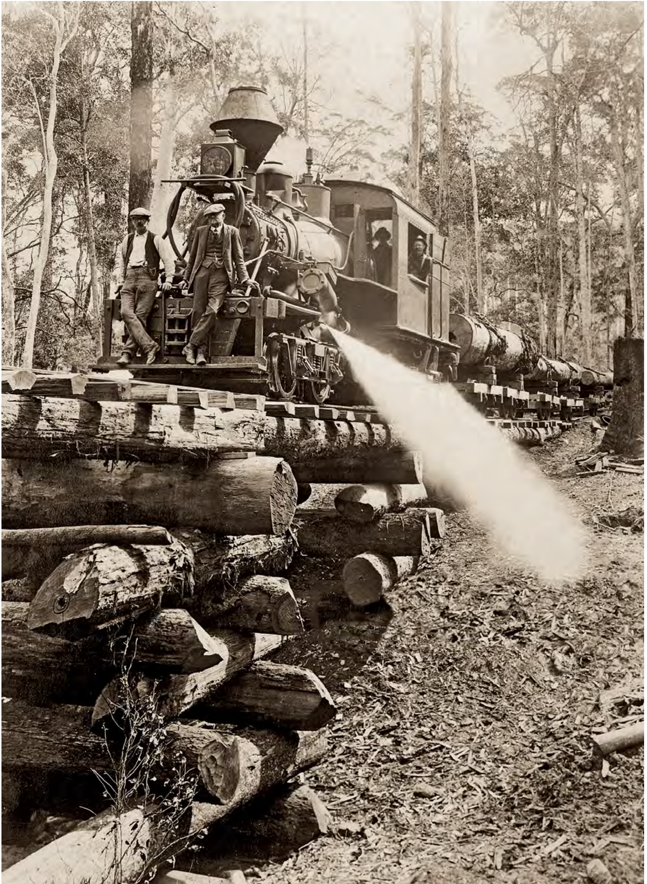
This fine image is one of a pair taken at the same location, believed to be on a recently constructed section of tramway along the Cataract Creek valley, west of Kendall. The date is thought to have been 28 March 1922. One suspects they are part of a batch of publicity photographs for Longworths' (Laurieton) Limited. Readers can see the other image on the back cover of Light Railways No.133, July 1996, available for free at: media.lrrsa.org.au/kabo133/Light_Railways_133.pdf Photos: Mark Plummer colln, LRRSA archives
