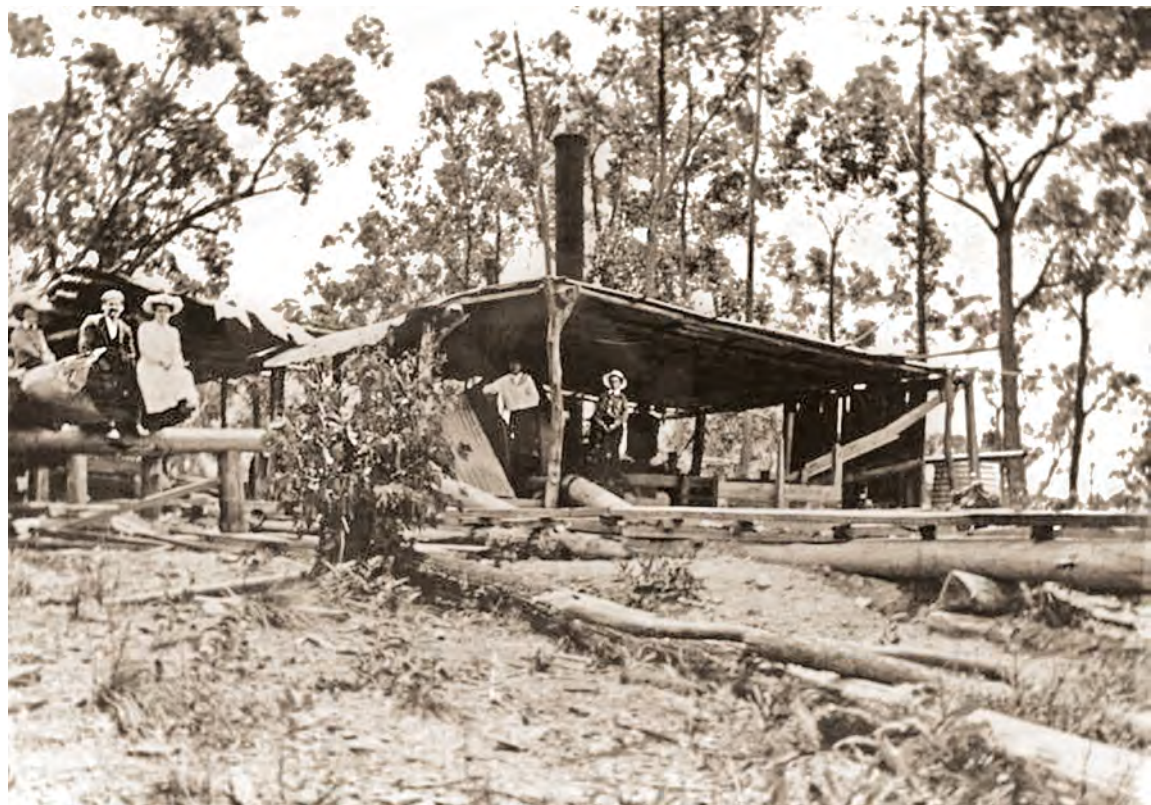
Joseph Tooth's 'River View' sawmill, c.1906. The mill was at this location for about four years, during which it was nearly burnt in the bushfires of January 1905. This was a favourite lookout spot for visiting tourists, being within walking distance of the Bundanoon station and village. Note the log tramway on right, about to head over the edge of the gorge, to the forest a thousand feet below. Photo: courtesy Bundanoon History Group
