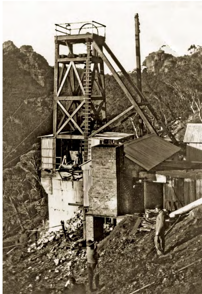
Owing to the increasing distance of the working areas from the No.1 and No.2 Shafts, adequate ventilation of the mine became a problem. In April 1930, construction of an air shaft, the No.3 Shaft, was commenced, two and three quarter miles to the north of the existing No.1 and No.2 Shafts. Completed in July 1931, it was initially used as an additional downcast shaft. In 1935, it became the main upcast shaft for the mine and the No.1 and No.2 Shafts became the downcast shafts. On 25 January 1952, a bushfire destroyed the headgear over the No.3 Shaft, which then collapsed into the shaft. The damage to the No.3 Shaft caused by the bushfire, and the underground fire in August 1953, led to the abandonment of the area of the mine beyond the site of the underground fire. The top of the No.3 Shaft was sealed on 19 October 1957. Photo: Lithgow Learning Centre
