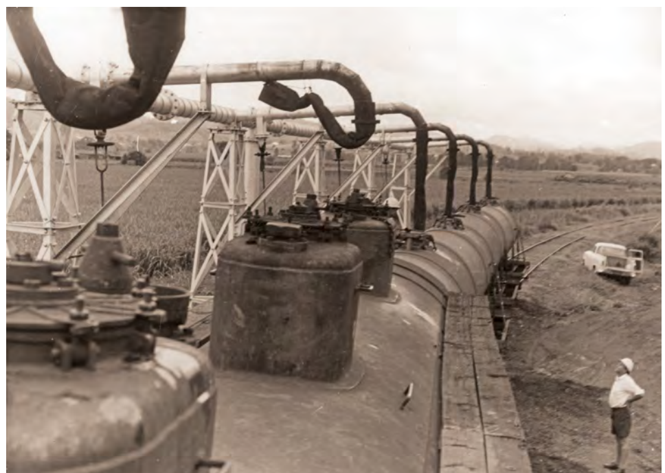
Condong's six-outlet molasses loader. This is on the Murwillumbah side of the then Pacific Highway level crossing outside the mill. TRMTH178-11
