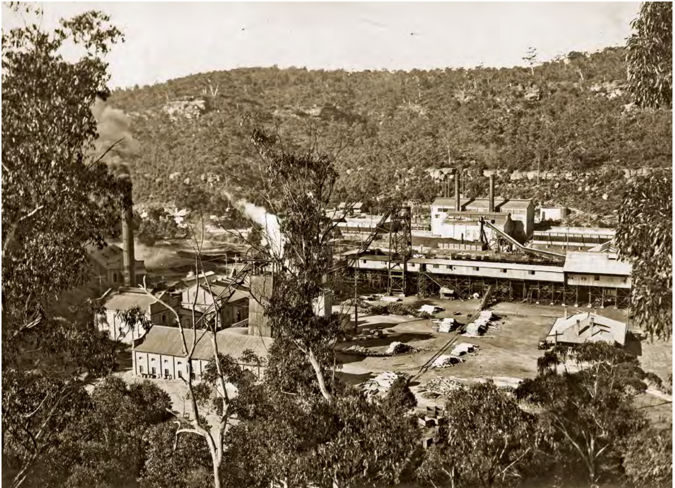
The State Mine in 1937, looking from the west. In the centre of the photograph is the headframe over the No.2 Shaft and the coal gantry. Above the gantry is the Lithgow Power Station. The power station was completed in December 1927 and was continually extended until, by 1937, it supplied power to Lithgow, Bathurst, Orange and Wellington. Modernised in 1949 and 1950, it was closed in 1960, when the Wallerawang Power Station was opened. When the Lithgow Power Station was opened, the mine's power house was de-commissioned and eventually converted into a bath house. The headframe over the No.1 Shaft is partially obscured by the tree in the middle of the photograph. In front of the No.1 Shaft are the stables. Photo: State Library of New South Wales, PXE 839
