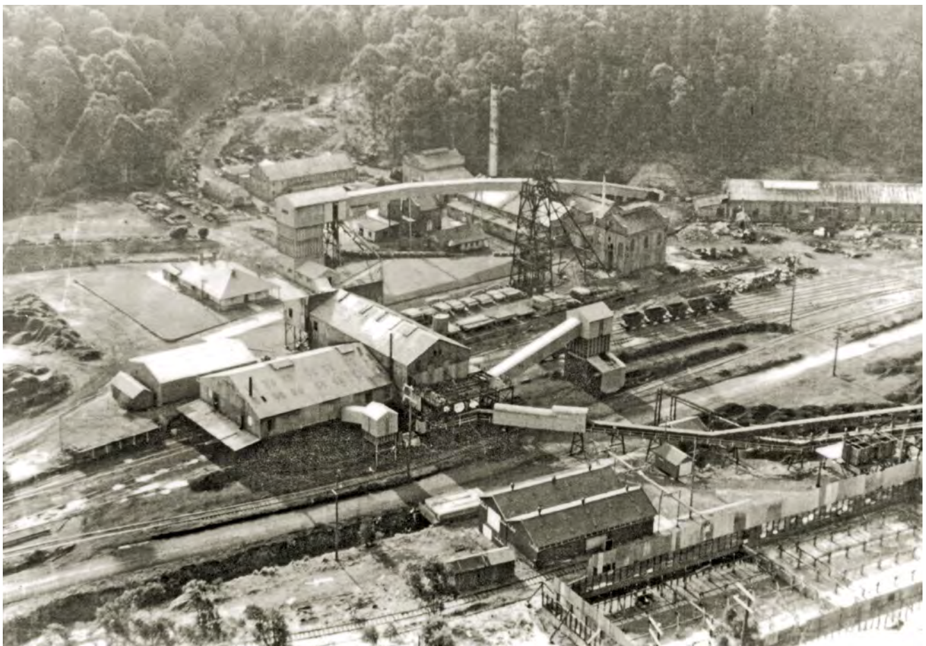
The State Mine after the completion of the new conveyor system in May 1959. In the right rear of the photograph is the workshop building and immediately to its left is the Middle North Heading Drift. The conveyor stretches from this drift, across the top of the bath house (original power house), to a storage bin. Only the headframe over the No.2 Shaft remains, as the headframe over the No.1 Shaft was removed in September 1958, to enable the construction of the conveyor. Coal winding via the No.2 Shaft ceased on the 22nd May 1959, and the gantry surrounding the No.2 Shaft headframe was removed. In the bottom right hand corner of the photograph, are the cooling ponds for the power station. Above the ponds is the conveyor for taking coal from the mine to the power station. Photo: State Mine Heritage Park Collection
