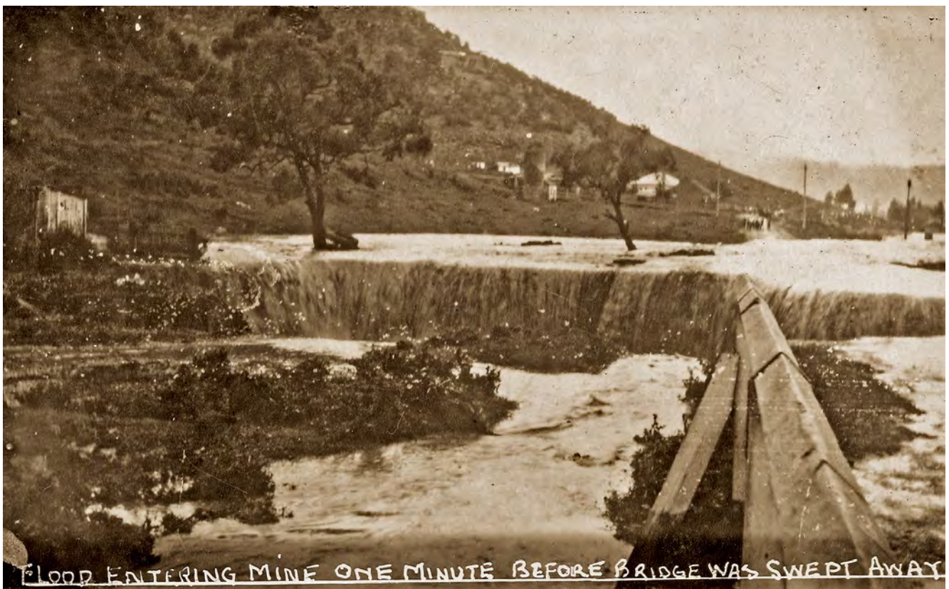
On the 19th February 1928, an intense rainstorm on the hills above Lithgow caused Farmer’s Creek to “become a raging torrent, sweeping over its banks.” The flow of water caused the roof of the Cobar Colliery to collapse and a cavity 100 yards in diameter was created. “The roar, as the earth subsided and the water rushed into the narrow neck of the tunnel was awe inspiring.” An estimated 175,000,000 gallons of water flooded the mine. A sandbag wall had to be erected to divert Farmer’s Creek away from the cavity, and months of pumping were necessary to dewater the mine. Fortunately, there was no one in the mine when the flooding occurred. The photograph shows the flood water entering the Cobar Colliery. When Farmer’s Creek again flooded the Cobar Colliery on the 10th June 1964, it caused the gradual flooding and eventual abandonment of the State Mine. Photo: Lithgow Learning Centre
