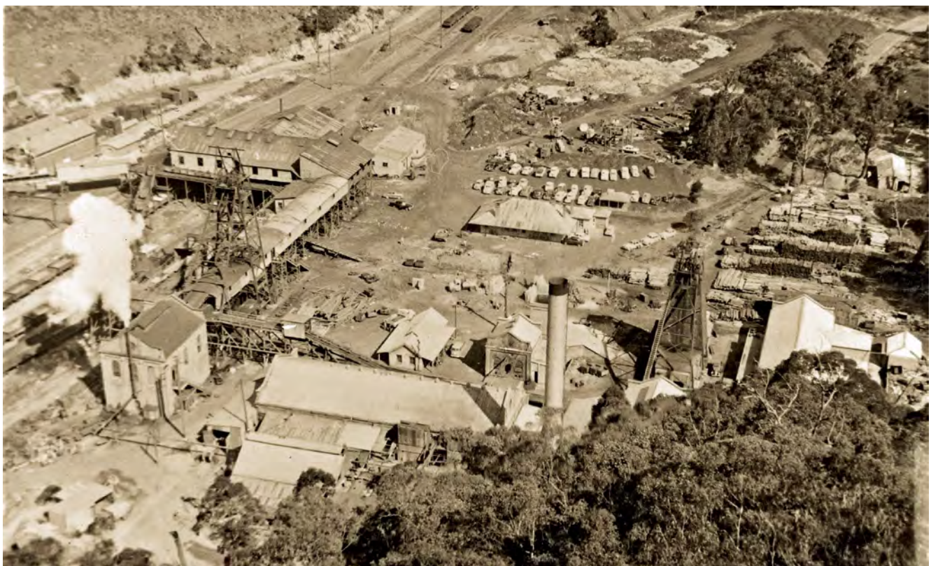
The State Mine looking from the north. On the left hand side of the photograph is the headframe over the No.2 Shaft. This was the coal winding shaft for the mine and it straddles the gantry that contained the tumblers for unloading the skips and the coal picking belts. On the right is the headframe over the No.1 Shaft, which was the mine’s upcast shaft, and to its left is the fan drift, fan house, fan engine house and the evasee chimney, which was used to expel the air drawn out of the mine by the fan. To the right of No.1 Shaft are the stables. Between the two headframes are the mine’s boiler and power houses. Directly above the boiler house chimney is the mine office. Photo: Department of Mineral Resources
