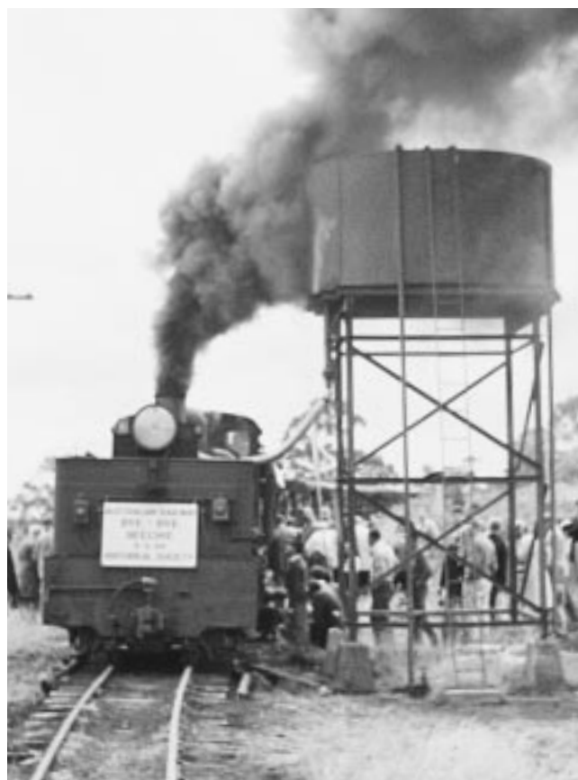
G42, at the head of an ARHS Special, pauses for water at Dinmont on 3 March, 1962. The steel water tank here, and another at Gellibrand, had been built to replace older corrugated iron structures only seven years earlier, an act which at the time must have given considerable heart to fans of the railway. Photo: Peter Charrett
