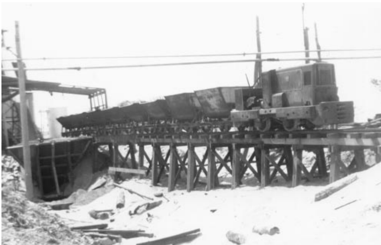
Ruston & Hornsby locomotive and skips on the elevated track beside the raw sand receiving hopper at the treatment works, 30 September 1955. Photo: Wal Larsen
