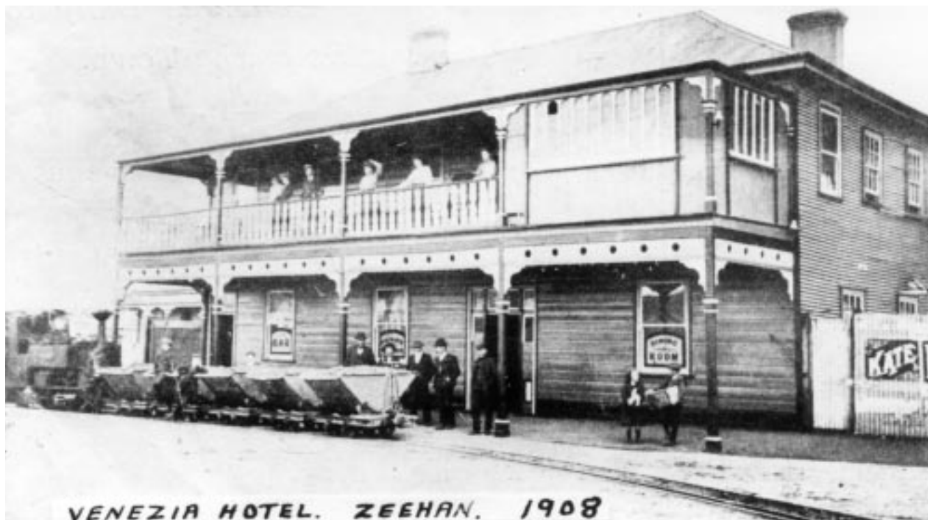
Western Mining Company's Black Hawthorn 0-4-2T locomotive WESTERN (1134 of 1898), with a train of side-tipping wagons, outside the Venezia Hotel, at the western end of the Zeehan Tramway Company's line in Main Street, Zeehan. The track in the foreground leads to Montana Loop. Photo: Zeehan Museum
