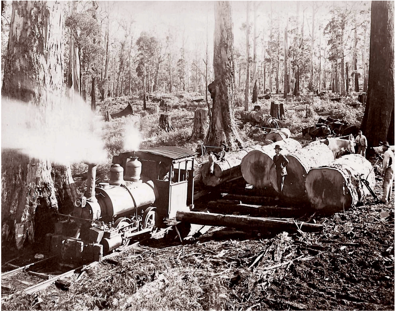
The Baldwin locomotive, at a log landing on the Comet Mill log tramway in 1898. Although showing the signs of 13 years of industrial use, at this time the engine still had most of its fittings. Of note is the lack of safety equipment in use by the workers and absence of protection for the engine crew from any excursions by the following logs. Photo: Australian Seasoned Timber Company album, Wandong History Group Inc.
