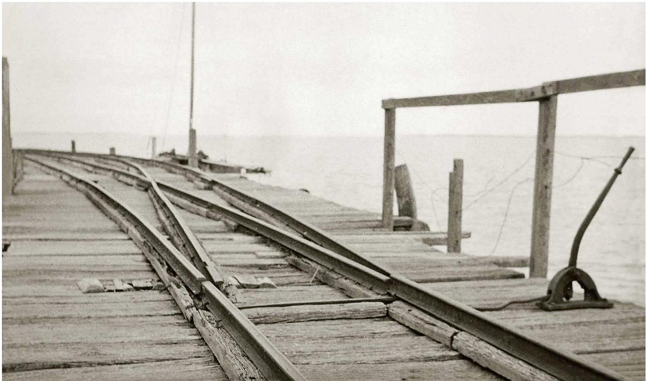
Close up of the stub points and track construction near the jetty 'elbow'. Note the rather battered point lever.
