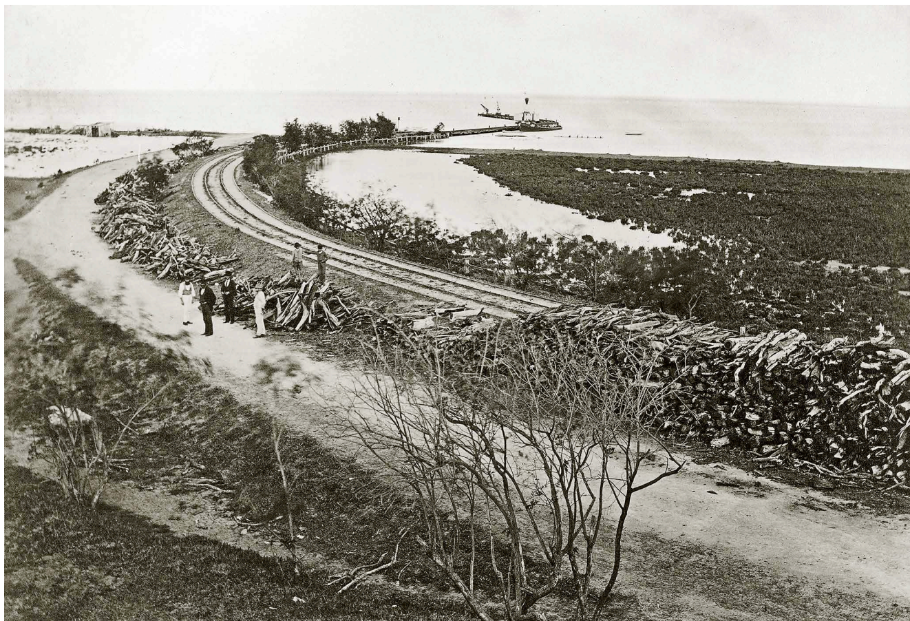
General view along the recently installed double track to the jetty, c.1875. From the base of the jetty to the elbow it was single track and then reverted to double track along the outer section. The new jetty crane plus the hand-operated travelling rail crane are visible. At left it appears drays have been dumping firewood billets which will then be stacked, ready for sale to the paddle steamers. The water level in the lake is at a moderately high level, inundating the samphire swamp and borrow pit for the embankment.
