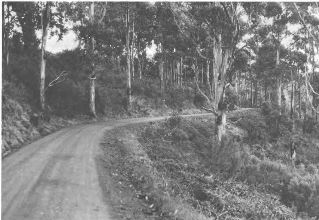
Easy gradients and sweeping curves, an obvious sign of an old tramway formation. This is the former Sandfly colliery tramway formation, now Allens Rivulet Road, 1 km east from Kaoota travelling towards Margate.
