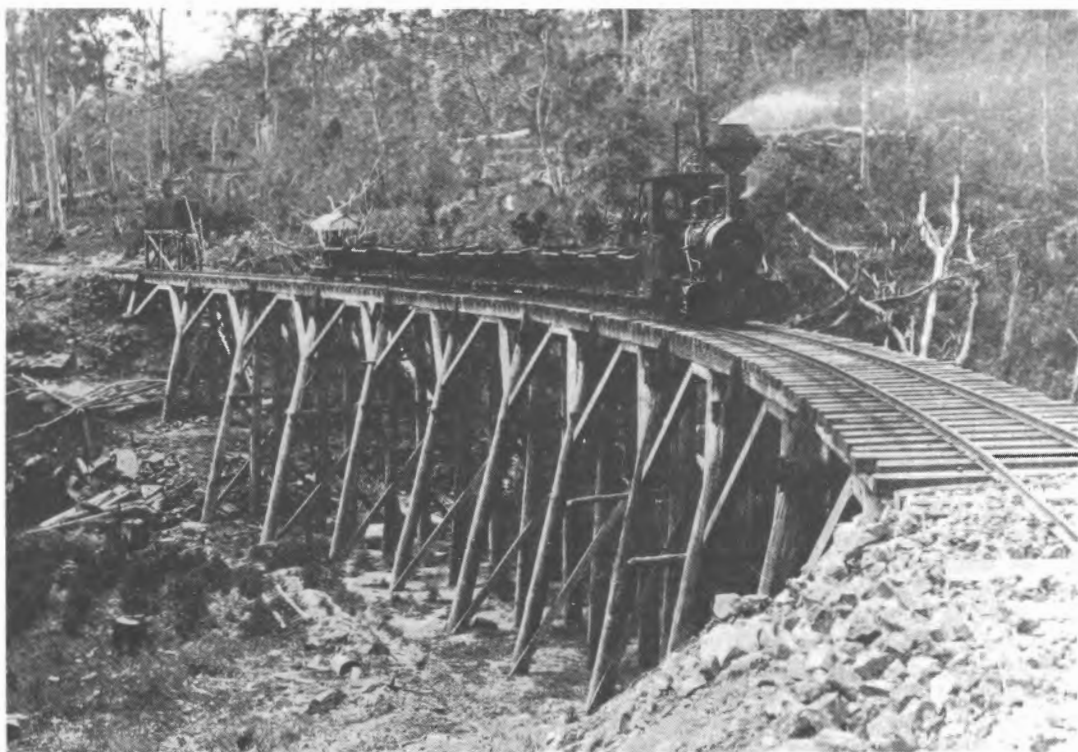
Krauss locomotive [B/No. 4526/1900] and empty wagons on the first bridge near Poverty Gully. Note the water tanks at the end of the bridge. Photo: Weekly Courier , 2 February 1907
