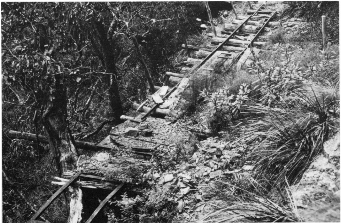
Endurance Mining Corporation: Syndicate tunnel tramway in Metz gorge showing skip turntable (April, 1982). Photo: R Mainwaring
