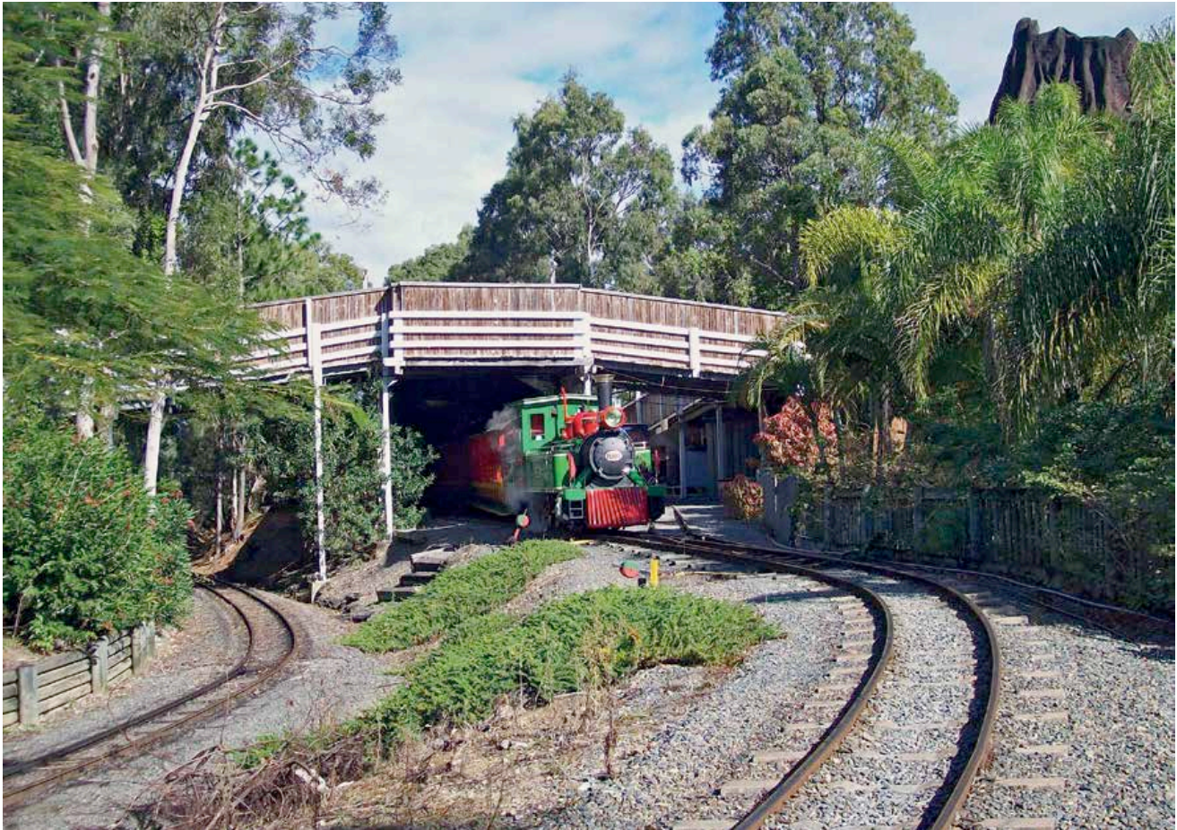
The scene approaching the Train Shed set in a secluded part of the grounds. The track to the left, at a lower level, is the main line at the top of the 1 in 40 climb, on a 15 metre radius curve. Photo: Teddy Hancox
