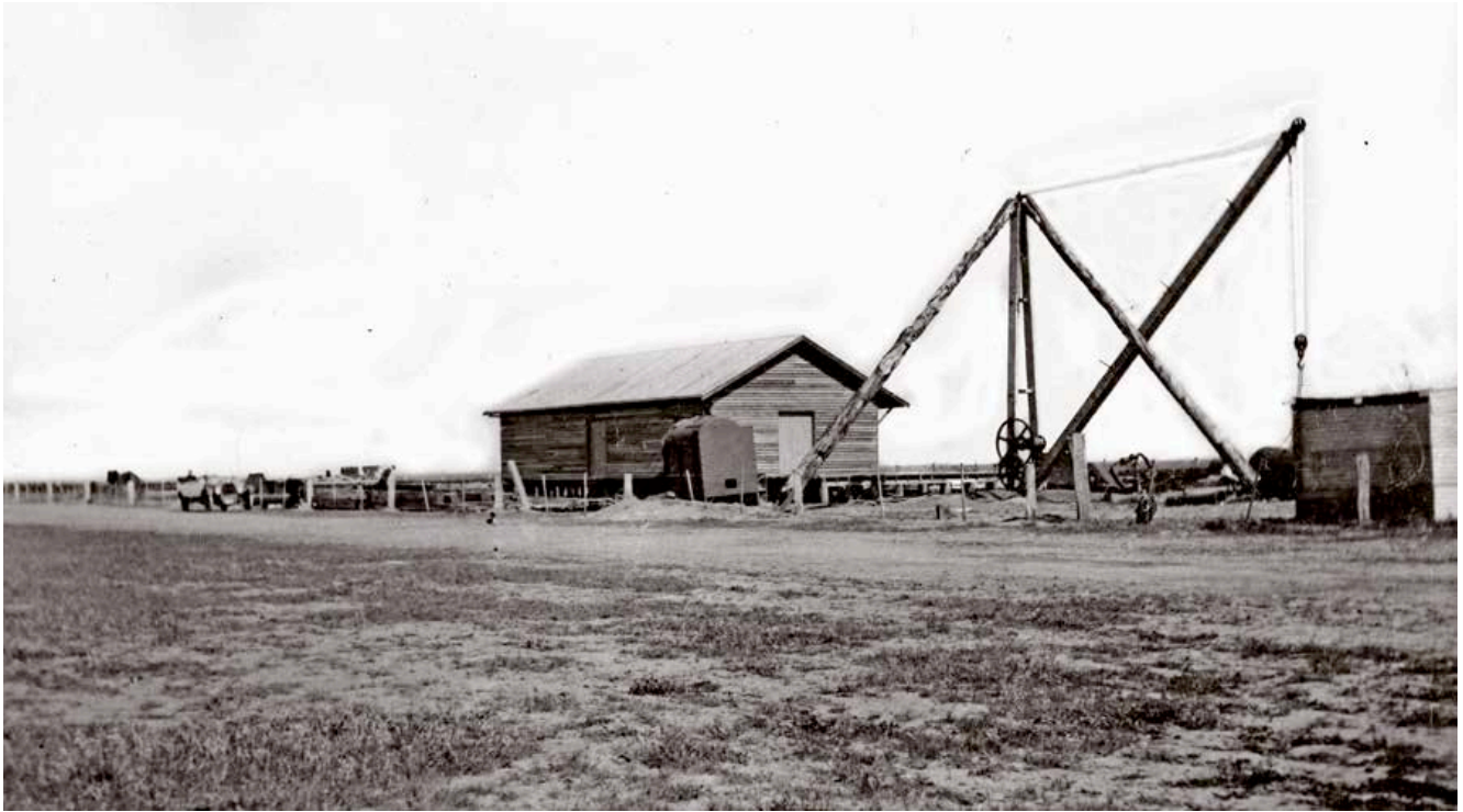
Torrumbarry Weir Siding c1921, prior to the installation of the tramway siding on the north side of the shed. Bags of cement, equipment en-route to the construction site, food and general goods were stored in the shed awaiting transport to the weir. The small structure on the right was used as an amenities facility for the workers at the siding and the train crews in between journeys. The image portrays the barren isolation of the area well.
