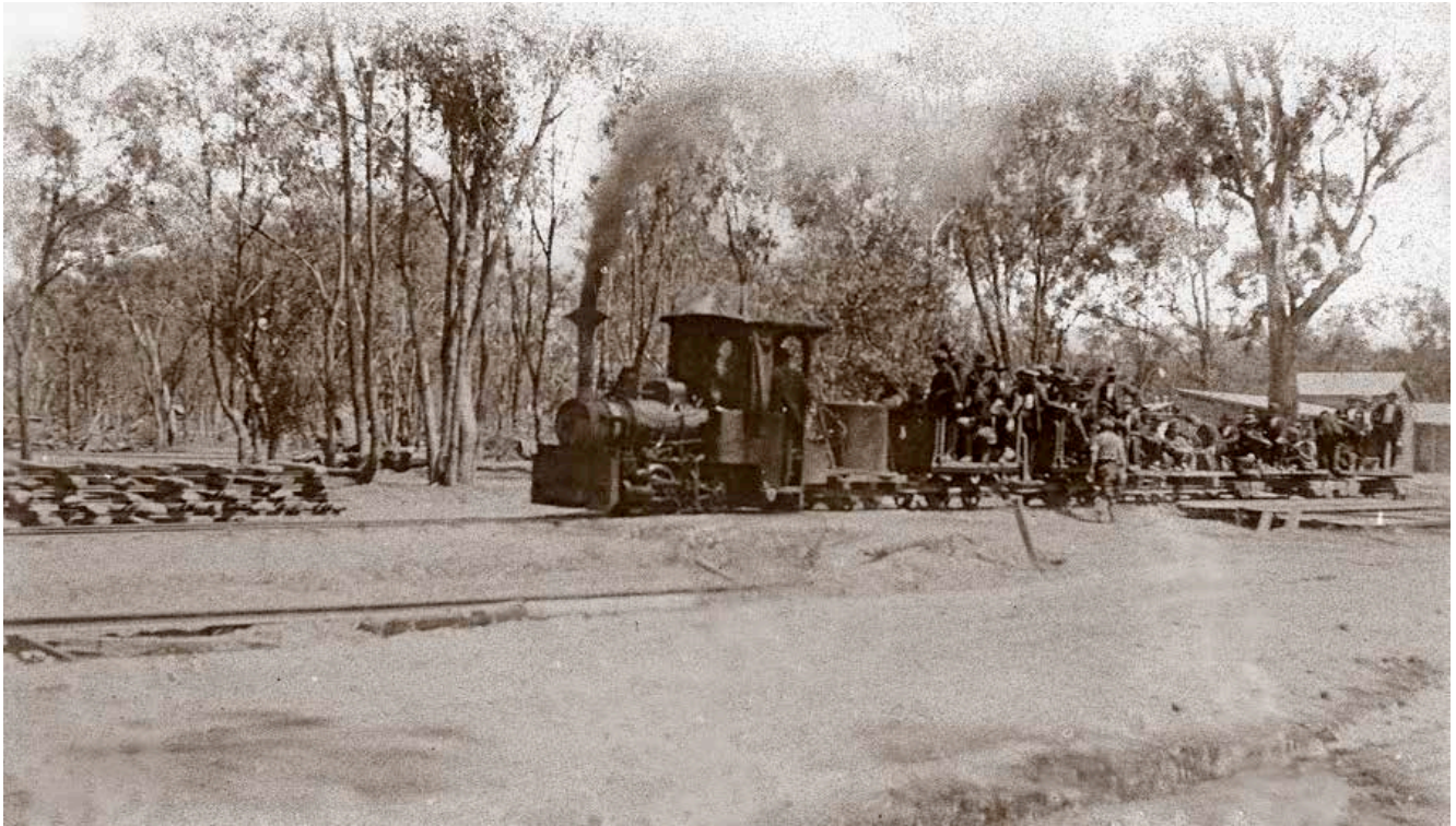
Another passenger train, this time hauled by Krauss, Robin, about to depart the weir site. The presence of a water tender behind Robin suggests that the railway siding was the destination. The Krauss was mostly used on short haul runs and did not usually make use of a tender.
