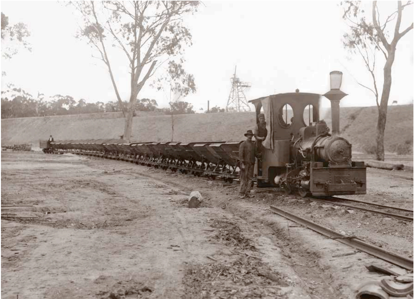
Krauss 0-4-0, B/N 2437 of 1891, Robin, returning from unloading fine sand, quarried from the bank of the Murray River, at Torrumbarry Weir and Lock construction site c1922. In the background, beyond the spoil bank, the radial tower, used to place concrete, is visible as is the 'guard truck', at the rear of the train. The occupant would assist with the shunting of trucks and the closing of gates along the way. Photo: State Library of Victoria
