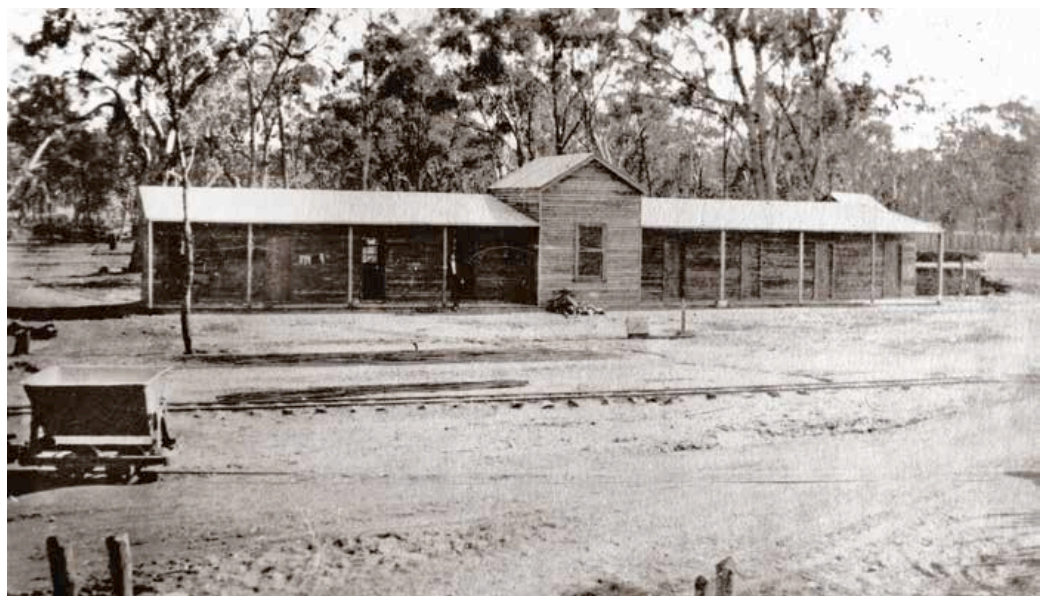
The officers' barracks at the weir site c1922. In the middle ground the main tramline to the hoppers, stores and workshops is visible while in the foreground the siding that served the sand heaps can be seen.
