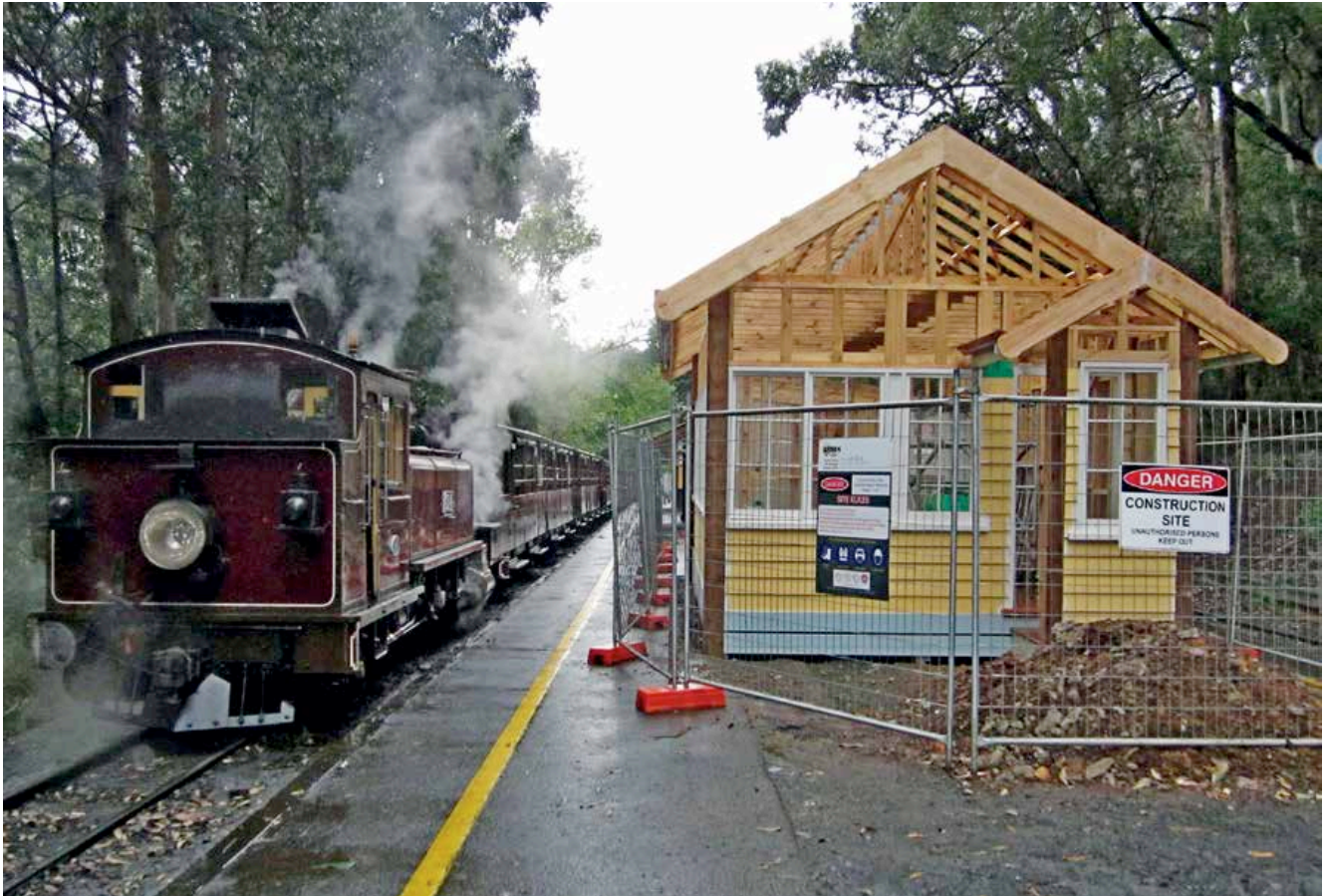
Above: The new signal box at the Puffing Billy Railway's Lakeside station in an advanced state of construction, 2 November 2018. Locomotive 12A waits to depart on the 1.30pm train to Belgrave on a wet Friday afternoon. Photo: Phil Rickard
