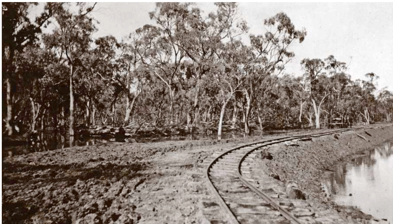
Probably taken on the access road to the weir (now Torrumbarry Weir Road) in 1920, not long after the tramway was completed and before gravel traffic commenced. The absence of any packing of the embankment made for a rough trip due to the uneven track. Photo: State Library of Victoria
