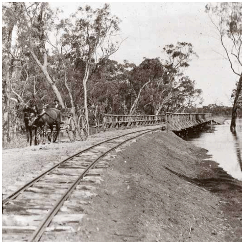
The only substantial structure constructed to accommodate the tramway was found around two kilometres from the construction site. The bridge over Cameron Creek was built to provide long term road access to the site. The flood prone country close to the weir site made necessary the use of a long embankment close to the weir site until the protection levee was reached about a kilometre north of this location. The rough-hewn sleepers and light rail were typical of most weir construction tramways. The absence of spilt gravel suggests a date around early 1920, soon after construction of the tramway was completed.
