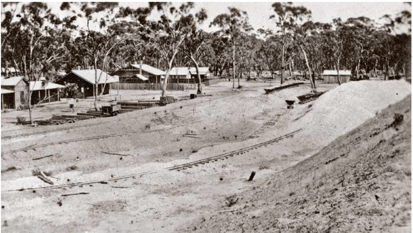
The sand and gravel dump site at the weir c1922. From the left can be seen the barracks, offices and houses for senior officials. The store yard for rail and construction timber was served by a siding, marked here by the small open wagon stored there. To its right is the main access tramway which travelled around to the hoppers, firewood mill and cement stores. Further to the right are the sidings serving the fine and coarse sand heaps and, evident by its lighter colouring, the Carisbrook gravel heap. The locomotive shed is visible at upper right. Photo: State Library of Victoria
