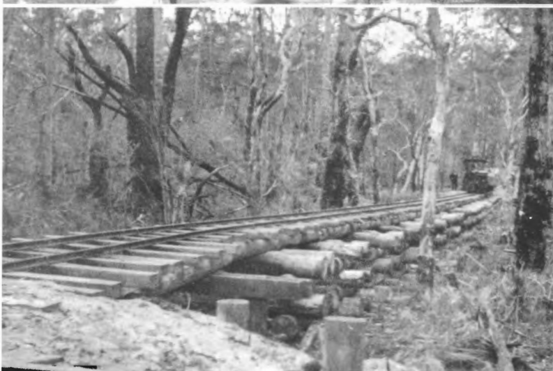
Posing for the photographer at knock-off time at the quarry loading point, c.1928. Photo: P Turnbull collection □ Deep in the forest, among the south coast gum trees on the northern section of the tramway, the Blackstone loco brings its train onto a wooden bridge built 'pig sty' style over a shallow depression. Photo: Newbold catalogue. □ The Blackstone locomotive and wagons on the wharf at Bannister's Point. Engineer Walter Islow sits on the running board, while engine driver Peter Carey leans against his charge. The loco appears to be in pristine condition. Photo: A McAndrew collection
