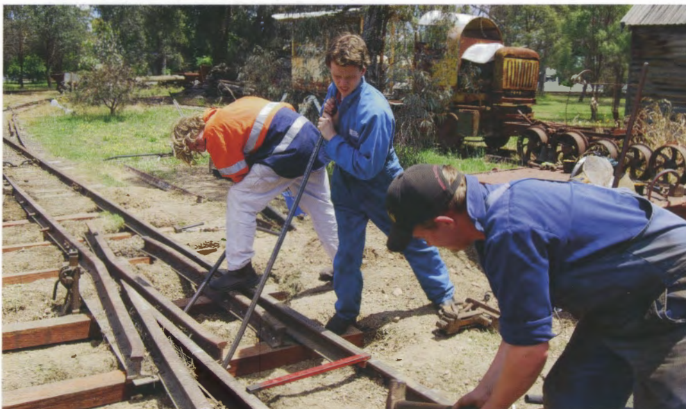
The track gang in action installing the new points in the main line at the Alexandra Timber Tramway on 30 November 2008. Photo: Peter Evans
