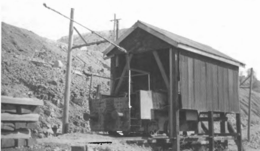
Mt Morgan Mine, 13th August 1957: abandoned 3ft 6ins gauge electric built on frame of Hunslet 0-4-0ST 796 of 1904, on Linda level. Photo: John Knowles
