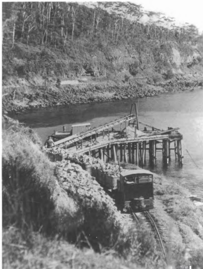
The Simplex bringing a load of silica up to the higher level at Bannister's Point. Note added inclined belt conveyor, silica stockpiled at grass beside the line and line of track discernable running along the foreshore in the background. Photo: A McAndrew collection
