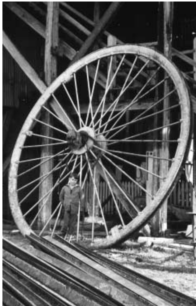
The author in front of the spare wheel for the downcast shaft headframe during 1960. The rails in the foreground were to be used in the Dudley Seam, but they were taken away and used at other collieries before the Dudley Seam was developed.
