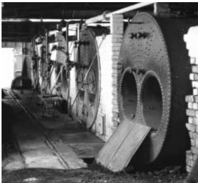
The bank of Lancashire boilers used for steam raising at the colliery. The skipway was used for ash disposal in the period up to 1930.
