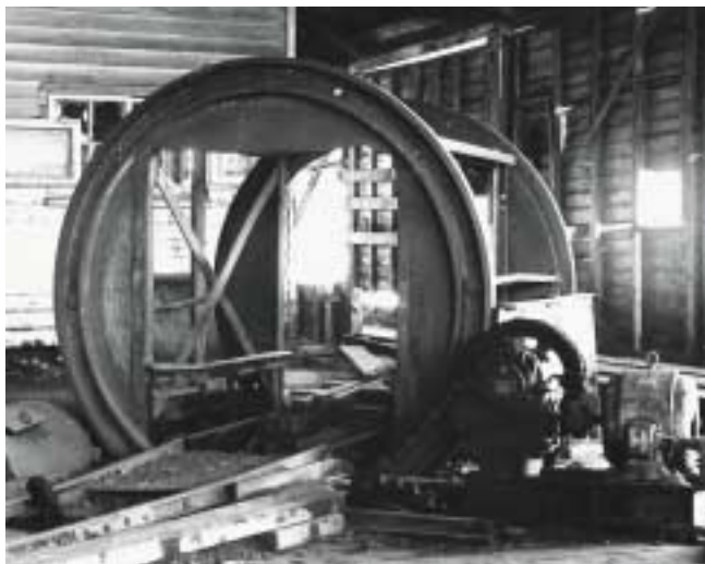
Very similar to the main skip tumbler at West Wallsend Extended was this example at Stanford Main No.2 Colliery. However, at West Wallsend Extended the driving mechanism was below floor level, a much safer arrangement. Photo: Brian Andrews
