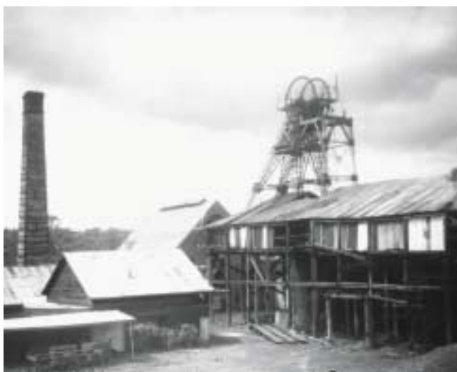
Taken from the embankment at bank level just after closure, this photo shows the heapstead. The sheeting on the building below the headframe conceals the skip tumblers and creeper. A couple of skips are to be seen by the shed at the left foreground, adjacent to a new cage frame which was under construction at the time of closure.
