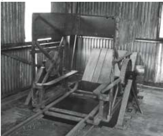
This end-tipping skip tumbler, similar to the one at West Wallsend Extended, was at Stockrington Colliery. Photo: Brian Andrews
