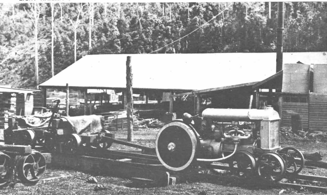
The first tractor which hauled log-laden jinkers from the forest to the mill, an altered 'Linn' tractor C1928. Part of the 'turntable' can be seen in the bottom of the photo.
