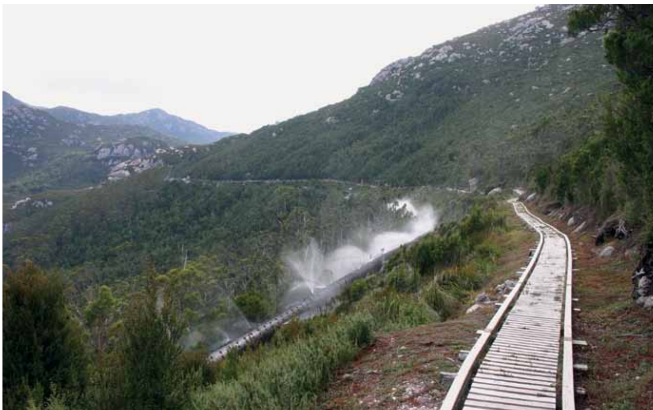
As if the West Coast rainfall was not high enough an additional ten per cent of precipitation, by way of spectacular geysers of Lake Margaret water, fell upon the bush land at many locations along the route of the original pipeline. Hydro Tasmania based its decision to close the Upper Power Station upon this unique spectacle. Lake Margaret itself lies just beyond the middle ridge. 17 February 2006. Photo: Nick Anchen
