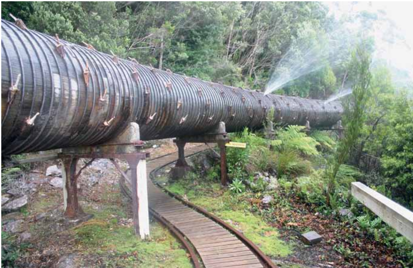
This location was known as 'the crossover' and is where the steel tram rails passed beneath the original pipe towards the lake end of the tramway. Headroom was very restricted hence the warning sign. The ferns are thriving from the copious leakage of water from the King William Pine pipe.
