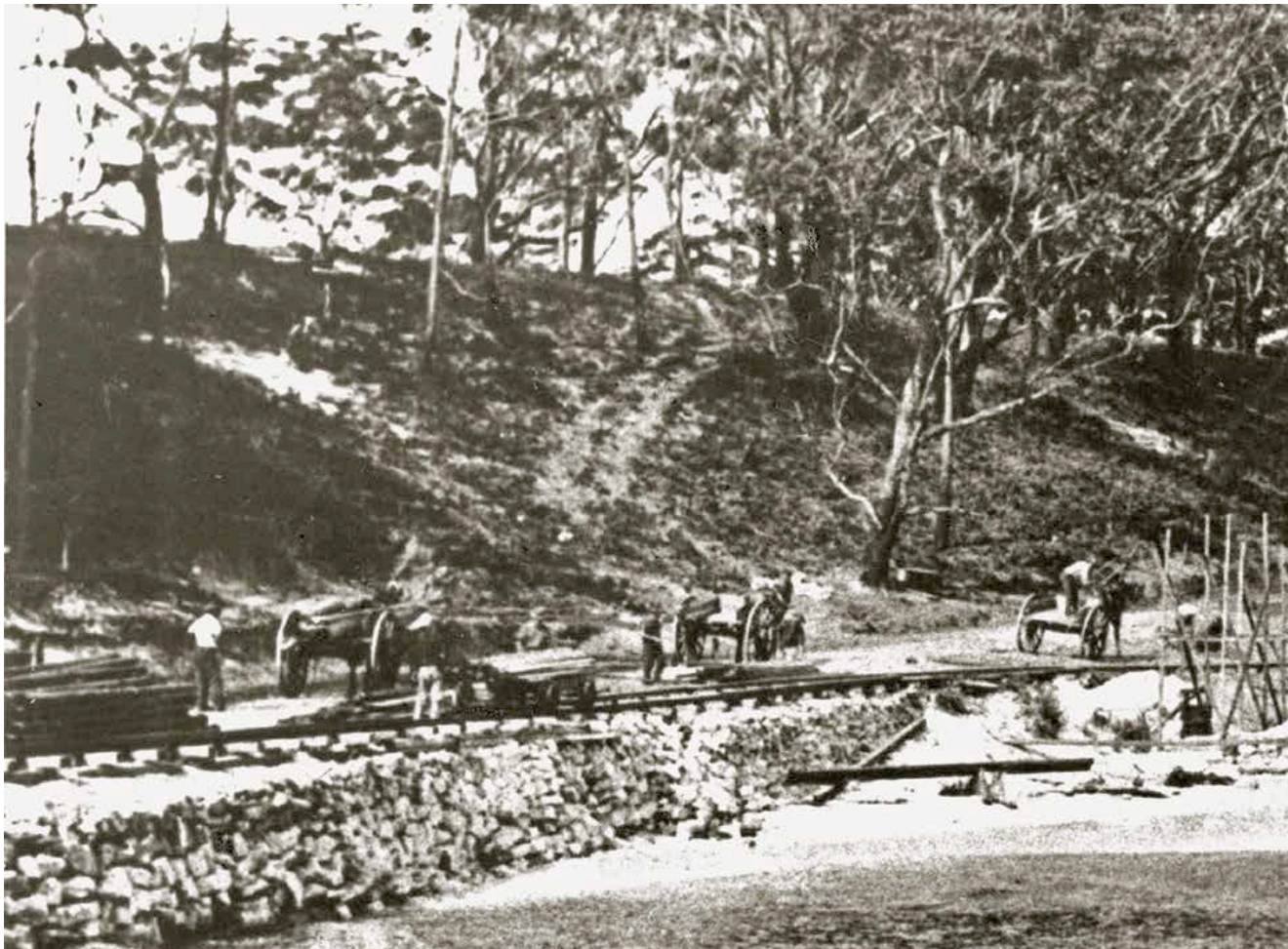
Seawall under construction. Date unknown.
