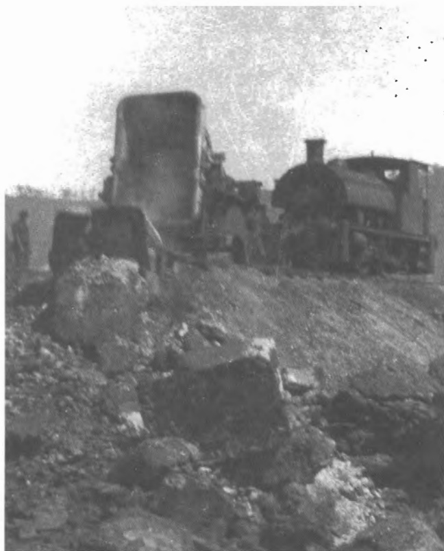
In 1926, Hawthorn Leslie 0-4-0ST WOMBAT (2658 of 1906) is dumping slag from the blast furnace, the task for which it had been specifically purchased by the steelworks' former owner, William Sandford Ltd. Photo: Grant McCarthy collection
