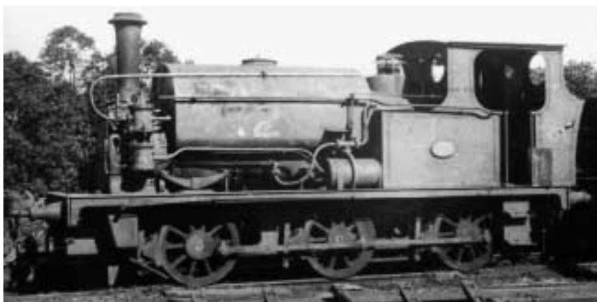
When its construction duties at Bunnerong were over, Hudswell Clarke 1530/1926 was fitted with conventional drawgear and air brakes, and put to work hauling NSW Govt Railways' coal hoppers from Botany siding to the power station. Photo: Bruce Macdonald collection, courtesy Richard Horne
