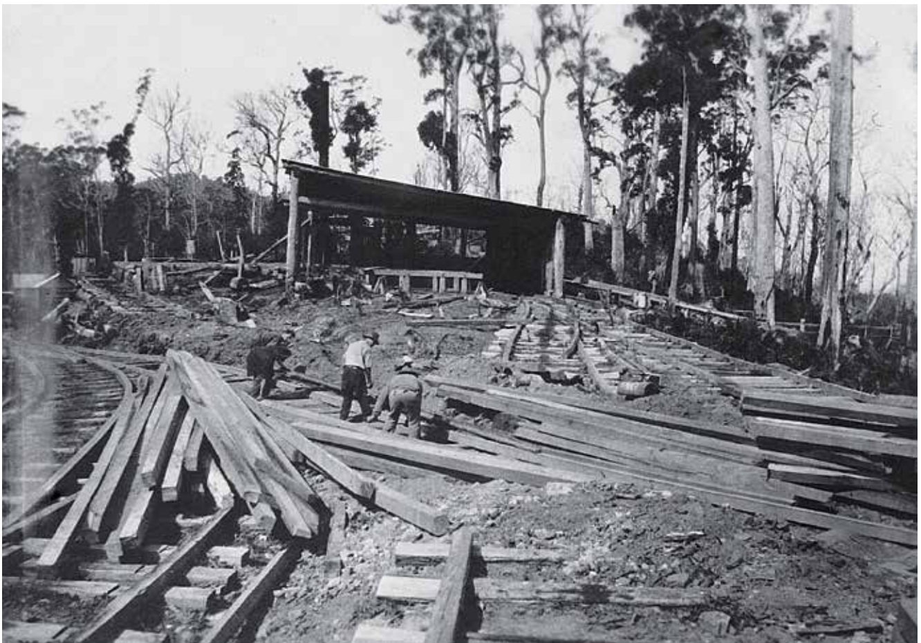
Constructing the Top Mill branch line on Knodingbal Ridge in 1932. The line on the left is the logging tramway going downhill to Mount George with a FWD lorry just visible in the background. The structure behind the workmen is the closed Rhodes Timber Company's 1927 bush sawmill. Its access sidings have been cut through by earthworks for the branch line. New wooden rails for the branch are stacked ready for laying.
