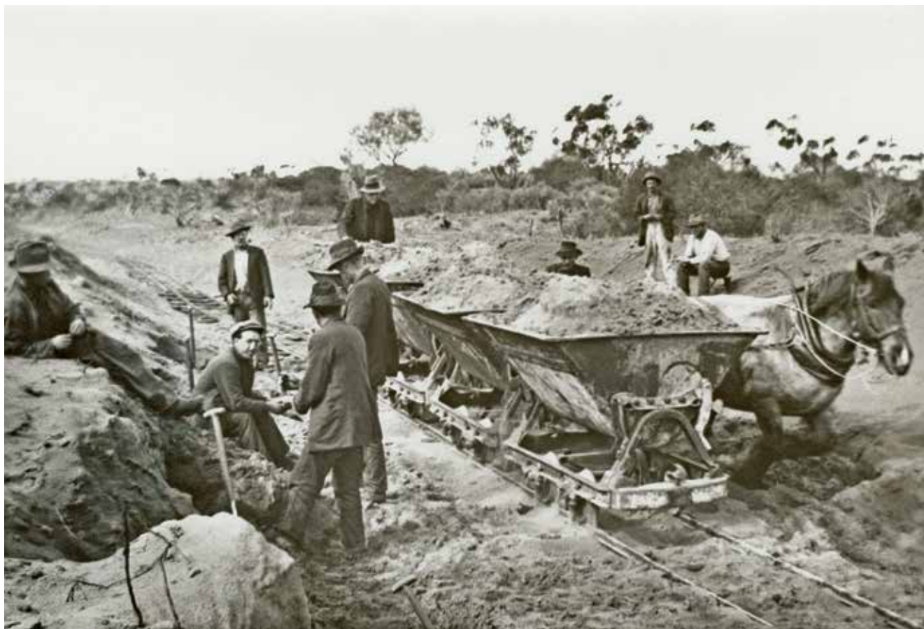
Side tipping skips are being used to remove the spoil from a cutting during the construction of the Trans Australian Railway. Whilst it is unknown where this photograph was taken, the sandy, scrubby terrain is exactly as found in the sandhill country east of Ooldea.
