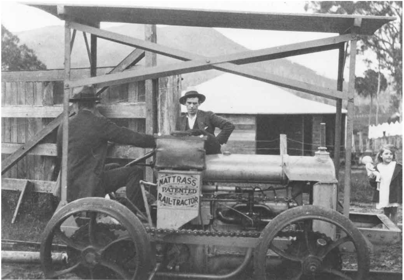
A Nattrass Rail Tractor, possibly at Mt George, though the presence of steel rails makes this uncertain. Weighing little more than 2 tons, the standard Nattrass was in essence a basic Fordson farm tractor fitted with railway wheels. The rear power take off provided power to the wheels of a permanently coupled log bogie. The resulting 8-wheel drive unit was exceptionally capable on rough and steep logging tramways. Rhodes Timber Company finished up with two Nattrass tractors and at least one home-made copy. Photo: Bruce Macdonald collection
