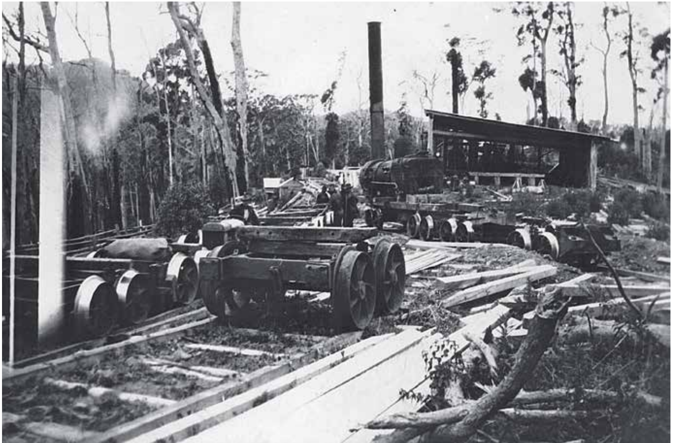
Preparing to rail the steam log hauler boiler to its new site at the end of the 1km Top Mill branch line. Judging by the bushes growing on the derelict Top Mill rail sidings several months have passed since the first photograph was taken. A Nattrass rail tractor with empty log bogies is sitting on the main line, while the boiler and an unidentified rail tractor are on the branch line. Photo: FC NSW 4 courtesy of Jim Longworth
