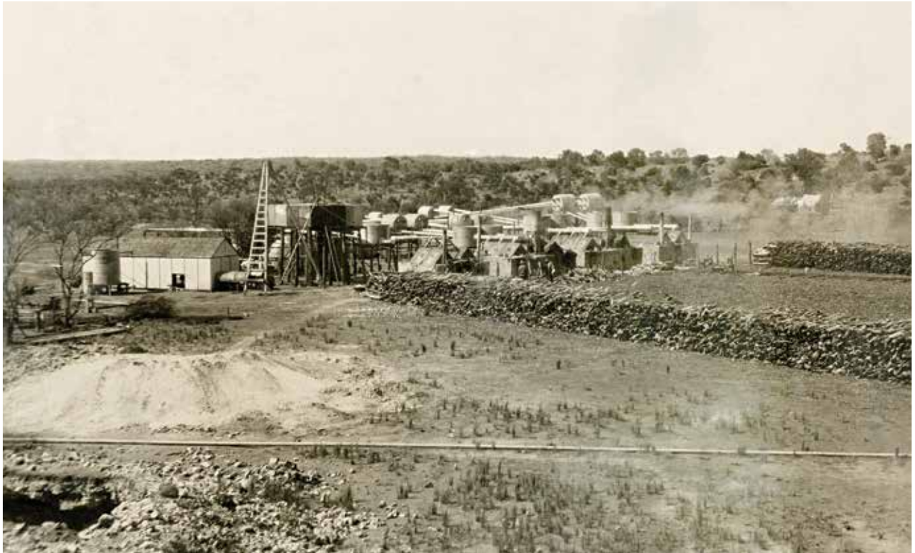
The 416½ Mile Condensers beside the ever-lengthening Trans Australian Railway. This slightly elevated view of the site, some 11 miles east of Ooldea, appears to have been taken from the embankment of the new line, just north of the site. It shows a busy scene of bore water being distilled into pure water. Saline bore water obtained at the site, was precipitated into steam in wood-fired condensers. This process separates salt from the saline water and once the steam re-condenses, the end product is extremely pure water, suitable for human consumption, not to mention eminently suitable for use in locomotive boilers. Long rows of firewood stacks can be seen on the right, and this is the firewood harvested south-west of the condenser location. It was brought into Ooldea on the 2ft gauge tramway and transhipped to standard gauge wagons to complete the journey. The location today can be easily recognised by rubble and rusting metalwork, and by a large stone and sand baker's oven. Photo: National Archives of Australia: B3104, Volume 4
