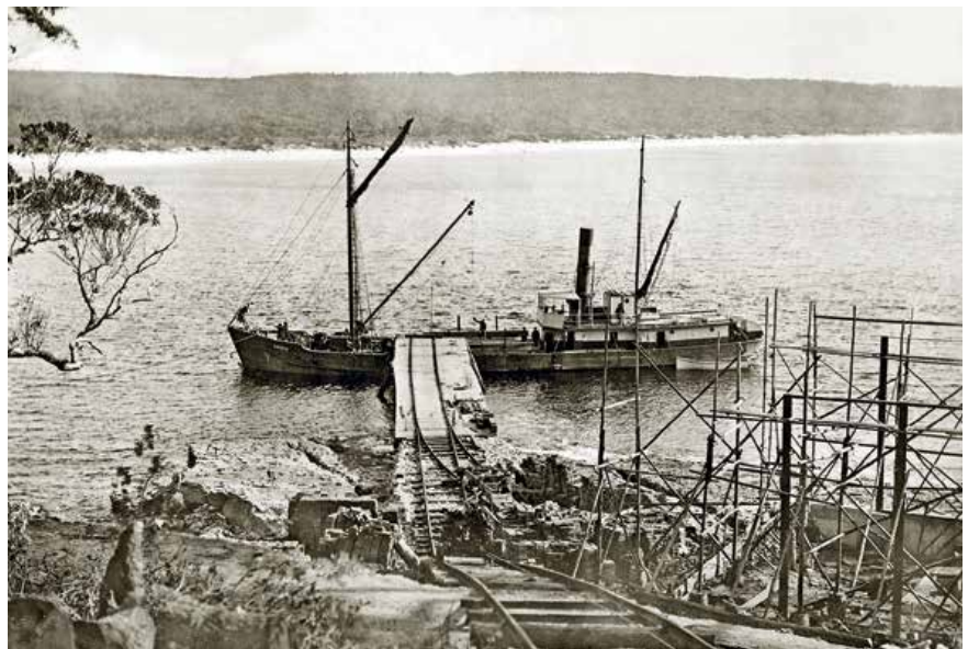
The ss Astral at unloading at the contractor's jetty. A truckload of timber is being winched up the incline; bricks are being unloaded from other trucks in the siding. At right, the power house is being built. (SLSA PRG 280/1/11/147)
