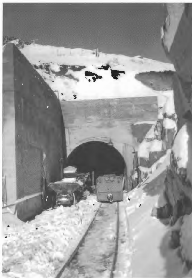
Snow scene. A Ruston & Hornsby locomotive at the completed outlet portal of the diversion tunnel in mid 1952. Its pristine condition suggests it may be the last one to be delivered. Alongside is a four cubic yard wagon and a Goodman-Conway Type 100 loader. The trestled portion of the spoil incline can be seen far up on the left hand side. NAA: A11016, 2110
