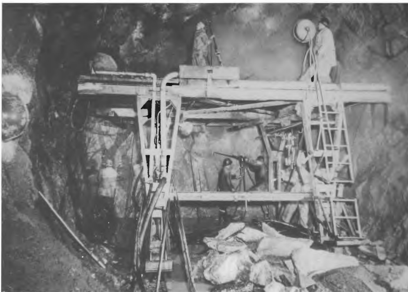
Drilling at the face from the two-platform jumbo using light air leg drills. Each miner would perform many tasks during each round of excavation. Photo courtesy F Selmer A/S
