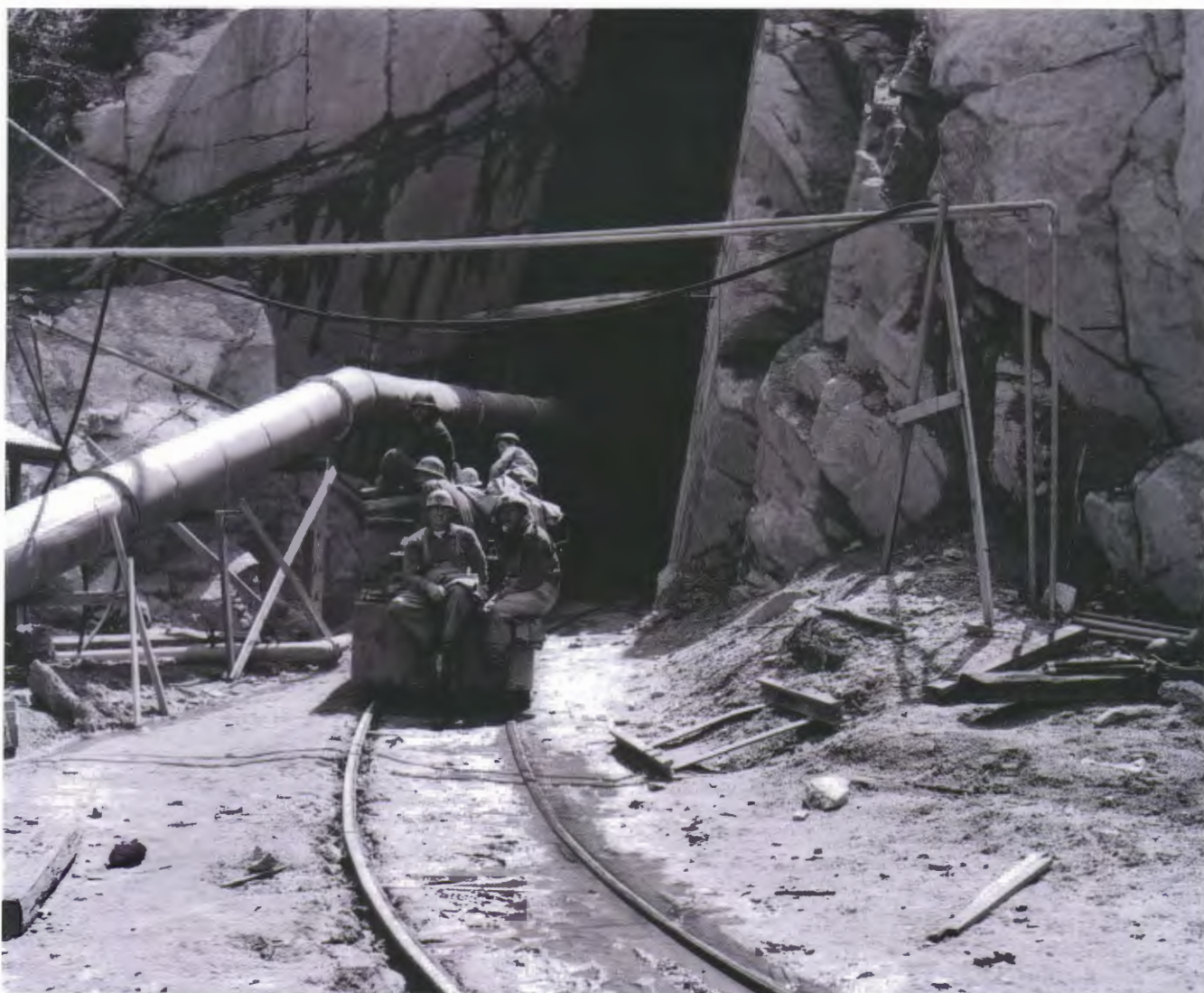
A Logan battery locomotive with a cargo of miners poses amid the sound rock of the adit entrance during 1953. NAA:A11016, 2997
