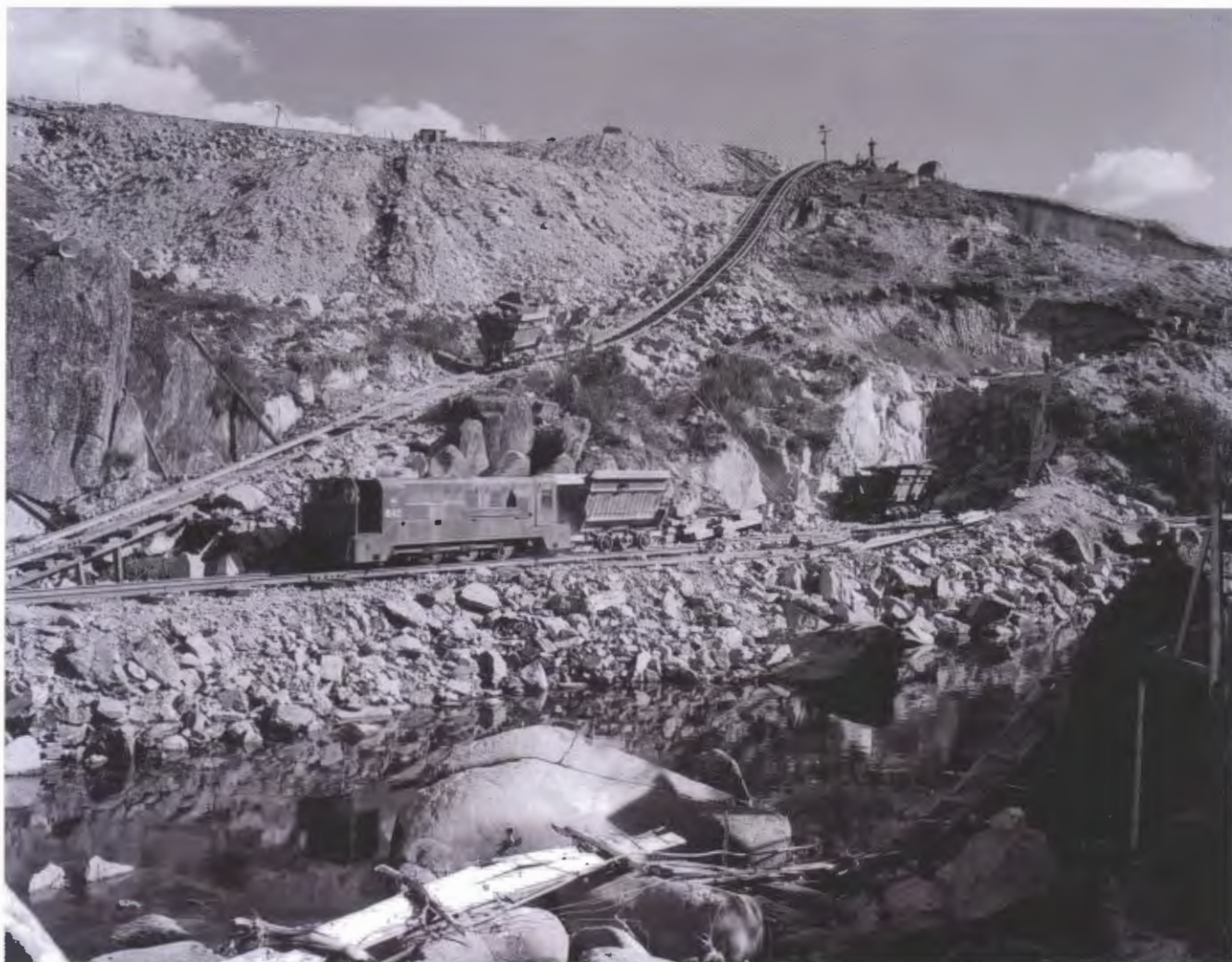
Ruston & Hornsby locomotive 13-C-2 at the site of the diversion tunnel outlet in early 1952. The photograph is taken from the bed of the Snowy River and the dam site is upstream to the right. A four cubic yard tipping wagon is being winched up the incline, with excavated material destined to be used in construction concrete.
