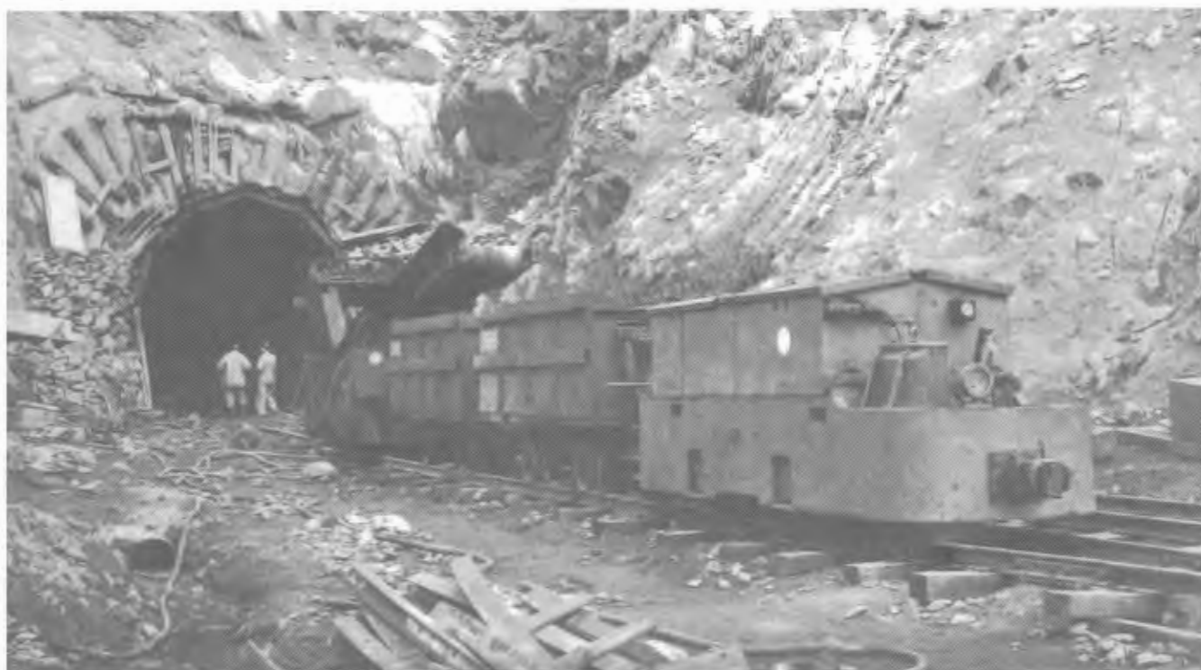
A Logan battery locomotive at the outlet portal of the pressure tunnel with a couple of 6-cubic yard Robert Hudson Granby cars and a Goodman-Conway Type 100 loader. The work required because of the poor rock at this portal can be noted. Author's collection
