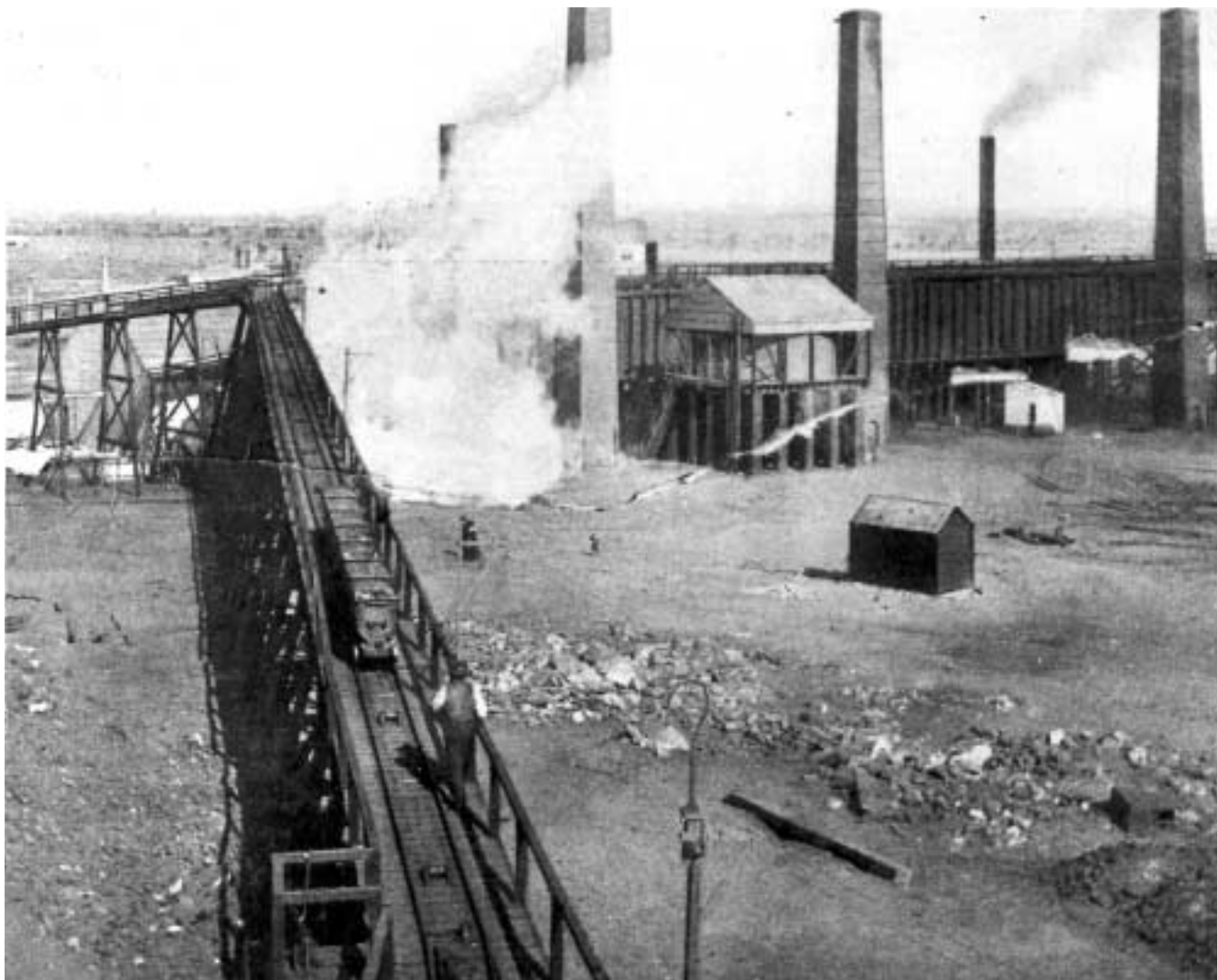
The rope haulage system was installed in 1905, to deliver the ore to the furnaces.
