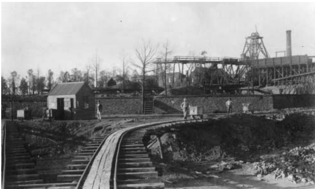
Hand-trucking ore to and from calcining heaps. Loaded trucks on the middle of the 'Y' are being weighed. Photo: Cobar Regional Museum
