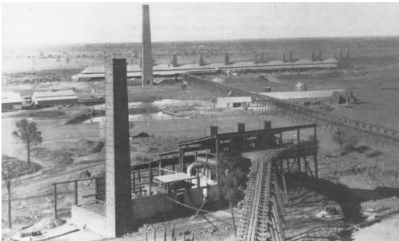
A view of the water-jacket furnaces in the foreground (c.1896), with the elevated tramway to the old furnaces in the background. Note the lower level narrow gauge line in the foreground for transporting coke to the furnaces. Photo: Cobar Regional Museum
