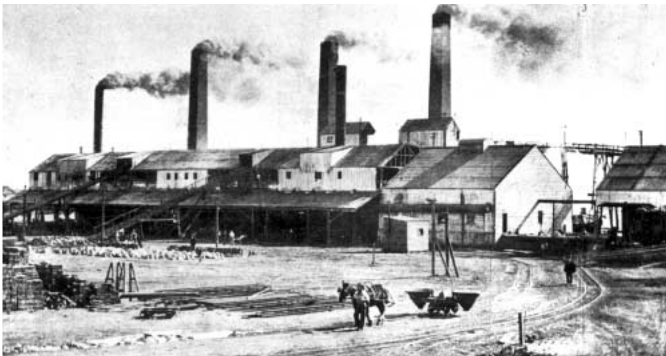
A horse hauling a Nasmyth slag ladle wagon from the furnaces, c. 1904. Locomotives replaced horses about this time.
