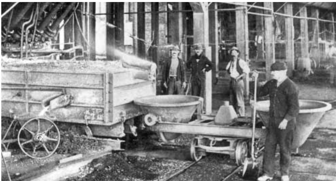
Pouring slag into a Nasmyth slag ladle wagon, c.1905.
